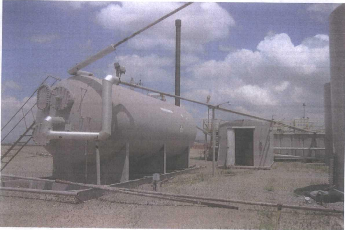
Chlorine Tanks & Air Compressor Shed
