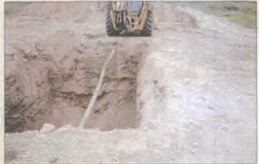
excavation & delineation 10 x 10 x 7-ft
