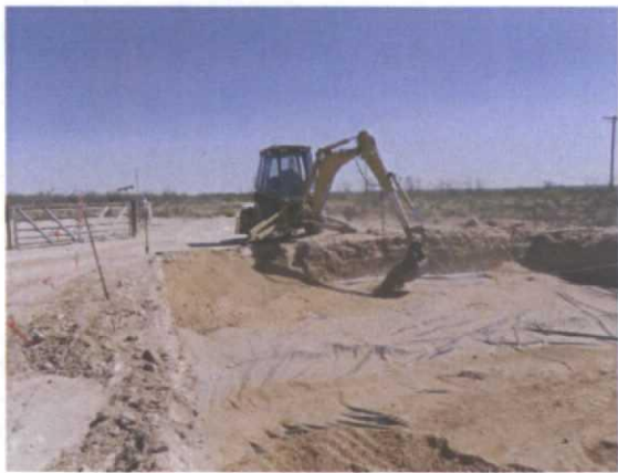
padding the liner with blow sand, facing north 5/17/2013
