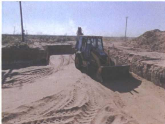
padding the completed excavation with 6 inches of blow sand, facing east 5/17/2013
