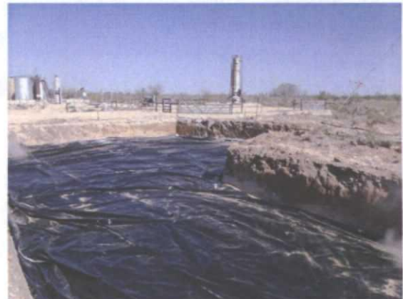
20-mil, reinforced liner installed at approximately 5 ft bgs, facing northwest 5/17/2013
