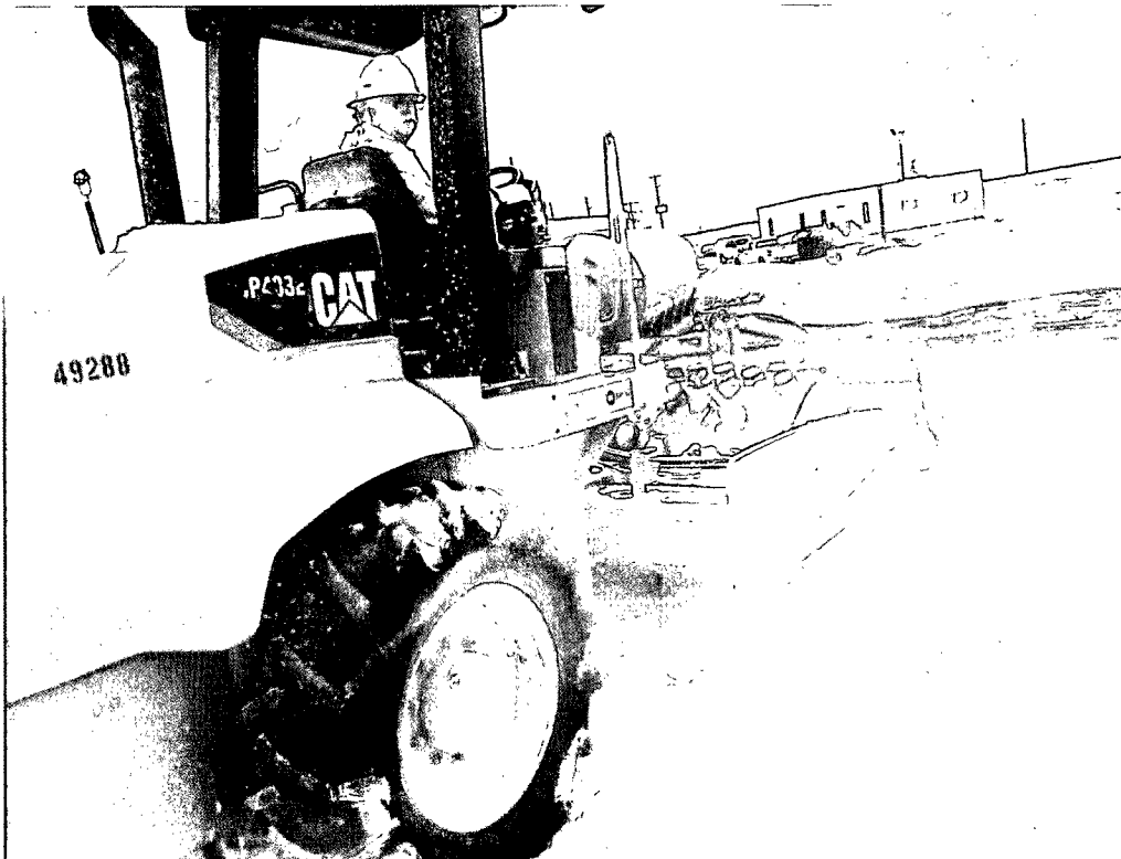
Compaction of caliche backfill, facing west 9/18/13
