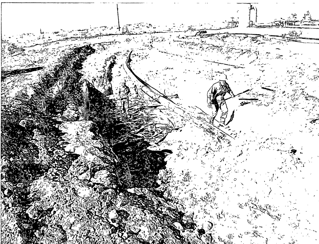
Photograph of the liner installation at the PLU #261/78 10" Mainline Release Site.
