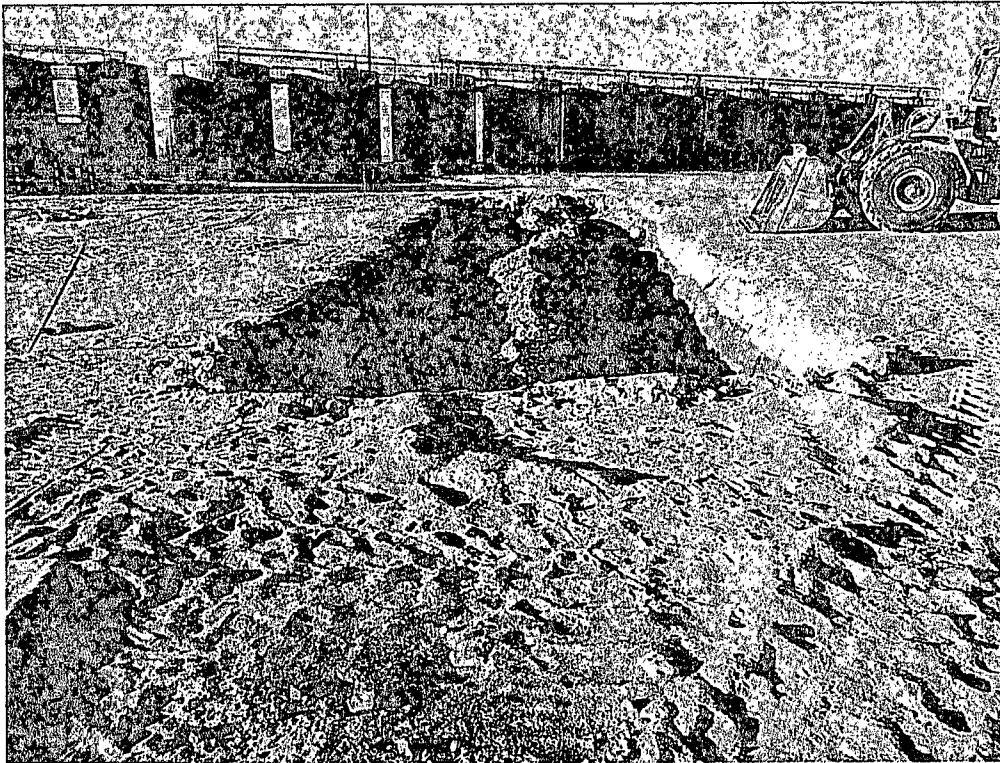
View Southwest – Excavation and clay cap installation in area of AH-7.
