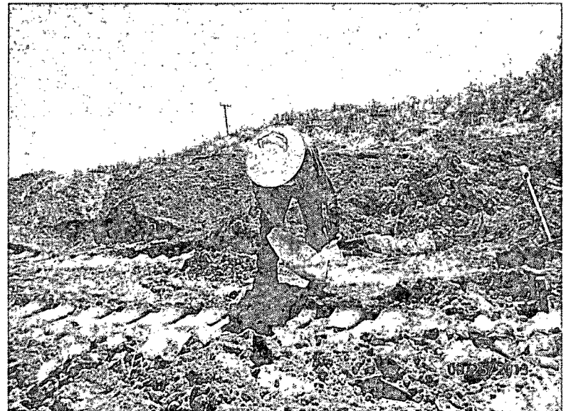
Plugging augur point in total with bentonite, facing south 9/25/13
