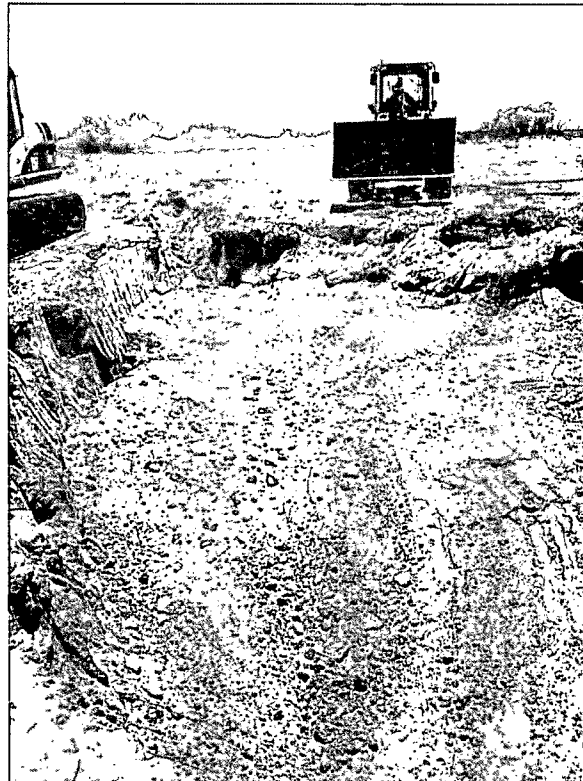
Photograph of the installation of caliche at the PLU #123 Illegal Dump Remediation Site.
