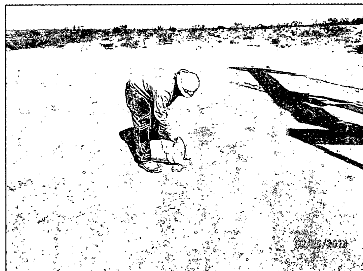
Plugging the augur in total with bentonite, facing east 2/26/13
