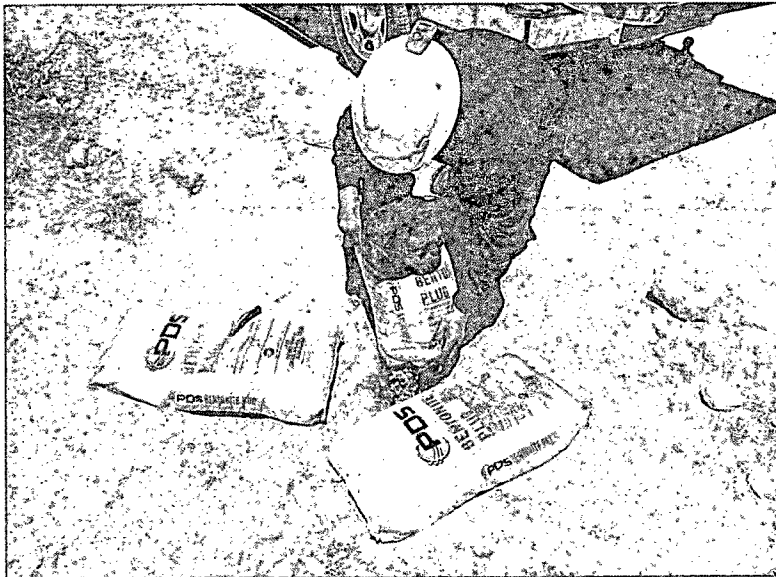
Plugging soil bore, facing north
