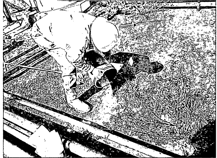
Plugging augur point with bentonite 11/1/13
