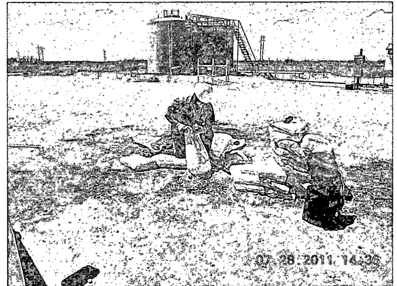
Plugging Temporary Monitor Well
