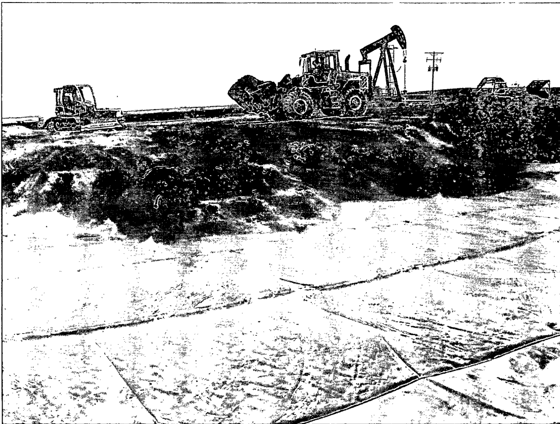
Photograph of the installation of pad sand atop the polyurethane liner in the southern portion of the well pad (Looking Northeast)
