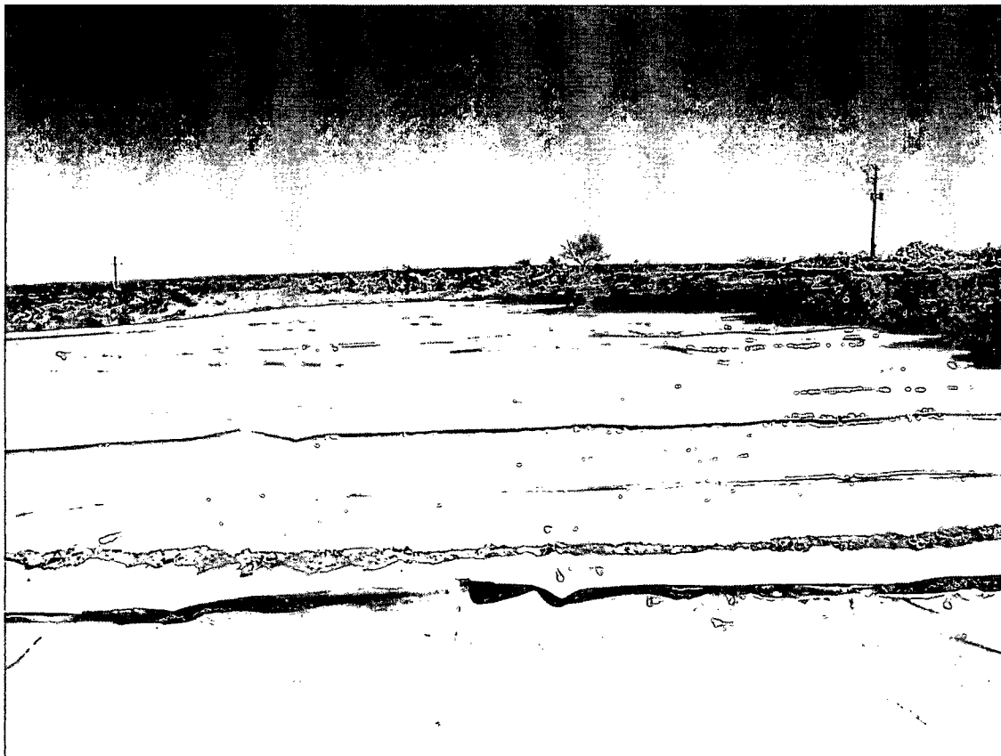
Photograph of 20-mil polyurethane liner cap installed on top of historic drilling reserve pit. (Looking East)
