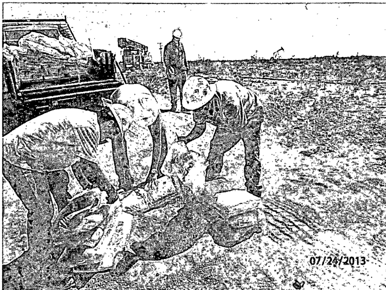
Plugging temporary monitor well in total with bentonite Facing northeast 7/24/13
