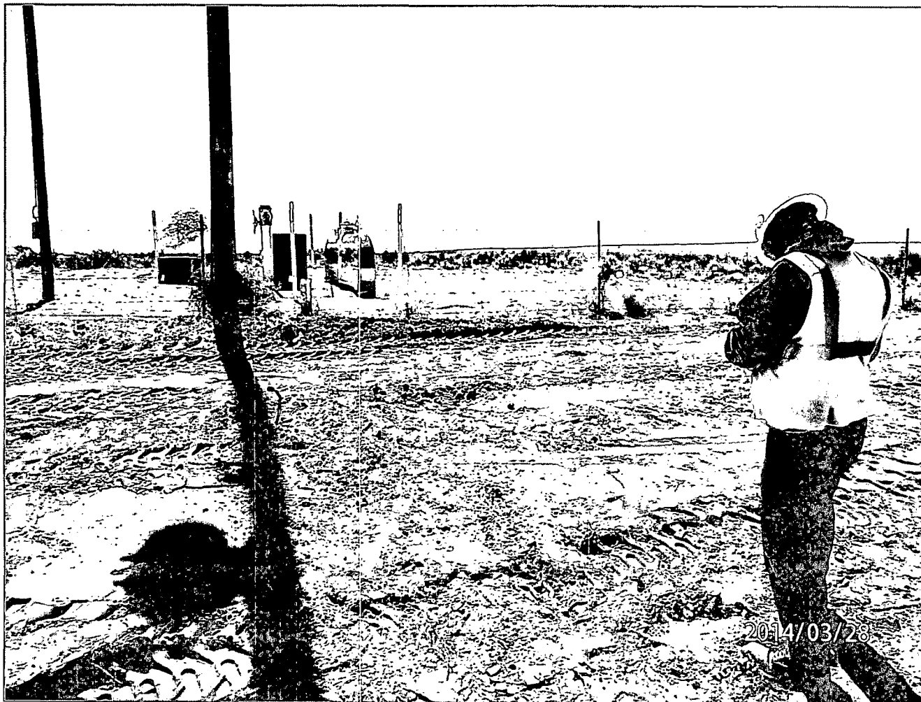
Impacted area along south side of County Road 7010 after excavation. Approximately 6" of top soil (~36 cubic yards) was removed from the release site.
