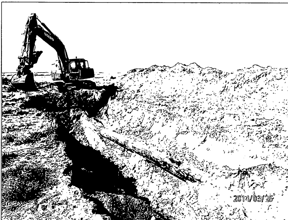
No evidence of contaminated soil upon completion of ~40' of exposed pipe.
