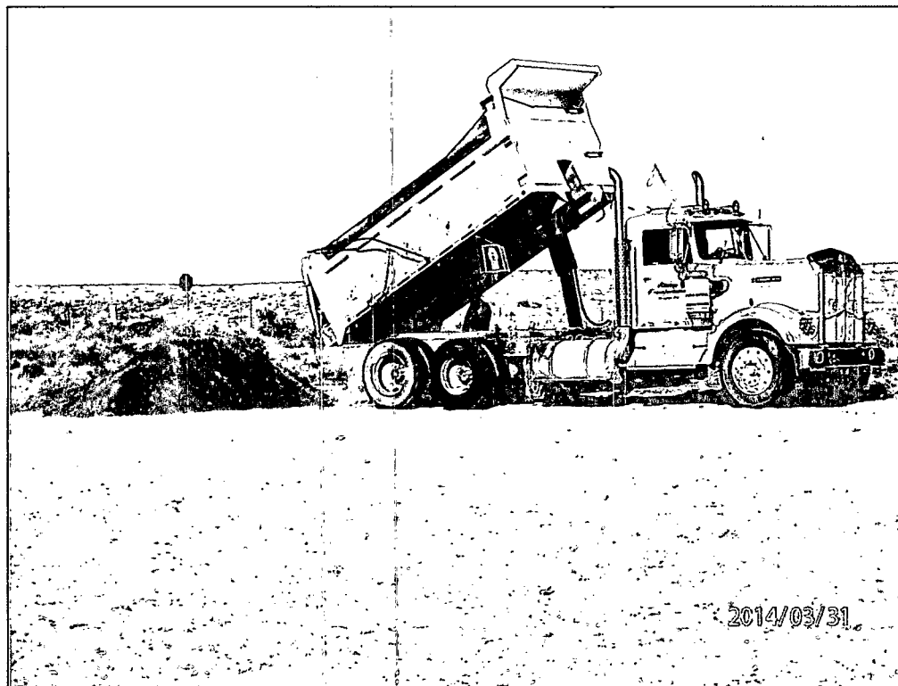
Off-loading clean soil for backfill of the pit. Trucks are also transporting the contaminated soil off location to the Envirotech, Inc. Landfarm for disposal.
