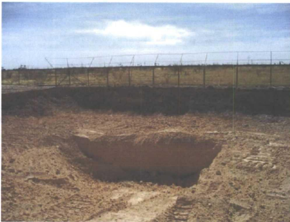
Concrete Removed and Vadose Zone Exposed for Inspection
