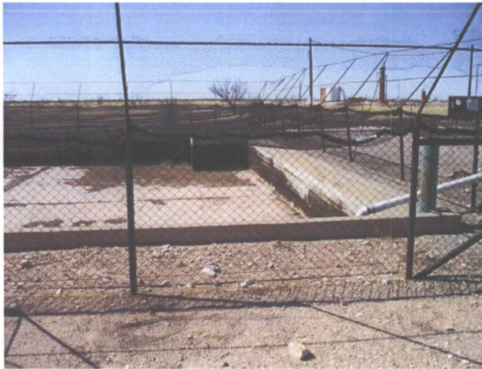
Drained Pit Ready for Inspection and Closure
