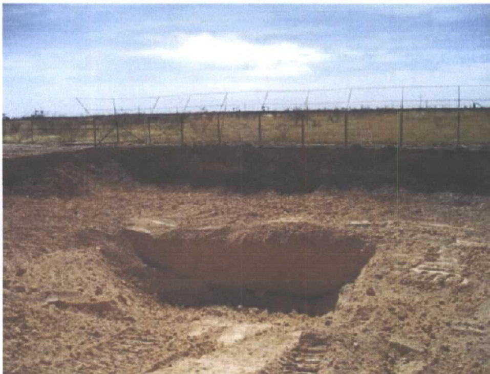
Concrete Removed and Vadoso Zone Exposed for Inspection
