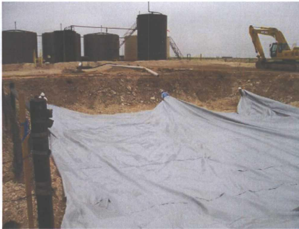
Liner Being Placed into Pit
