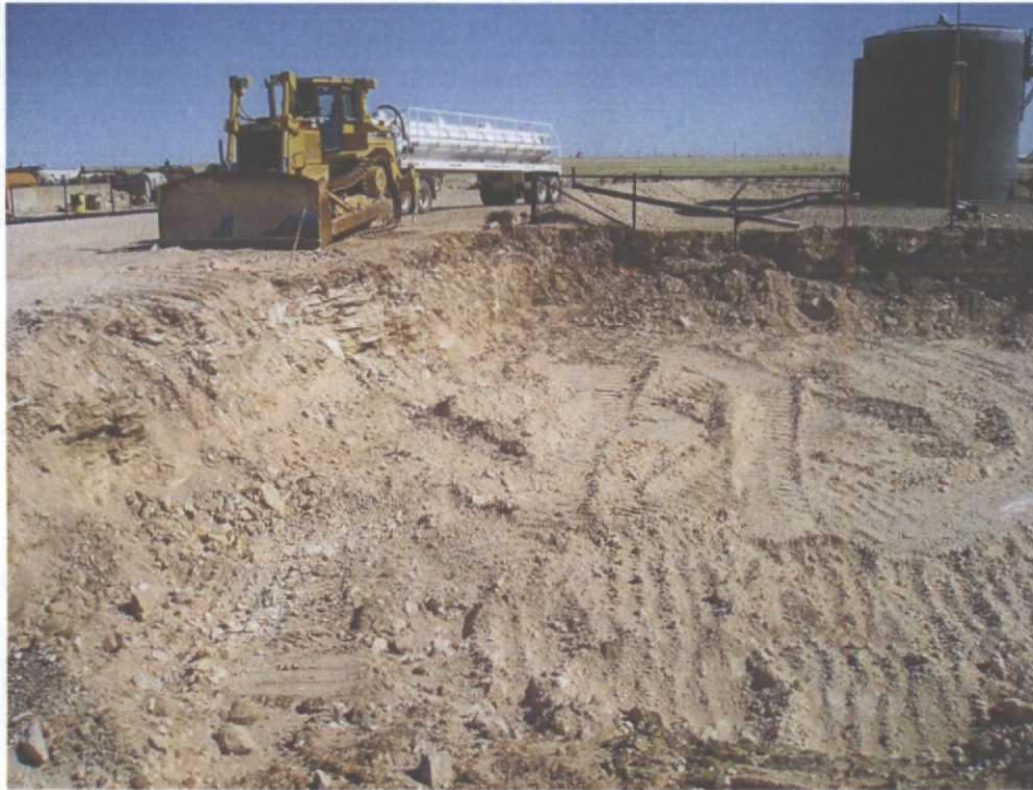
Pit Closure Following Concrete Removal
