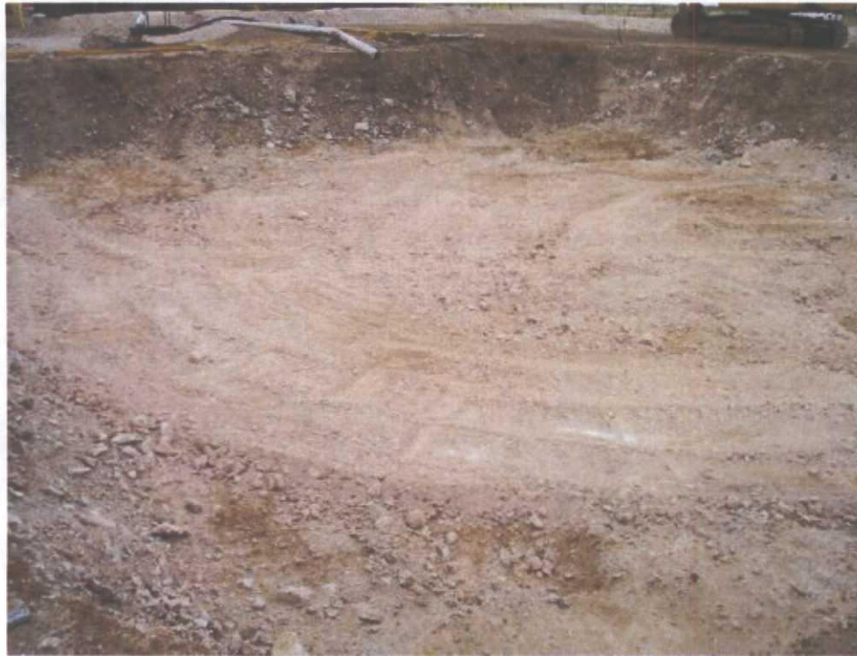
Pit Prepared for Liner Installation
