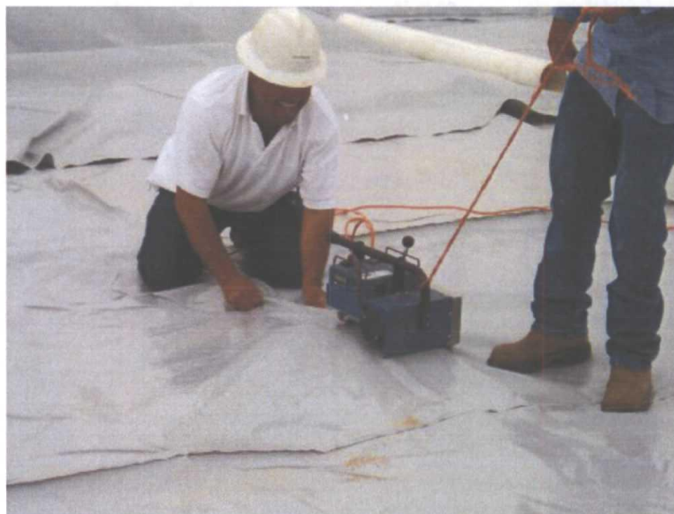
Seaming Liner for Installation
