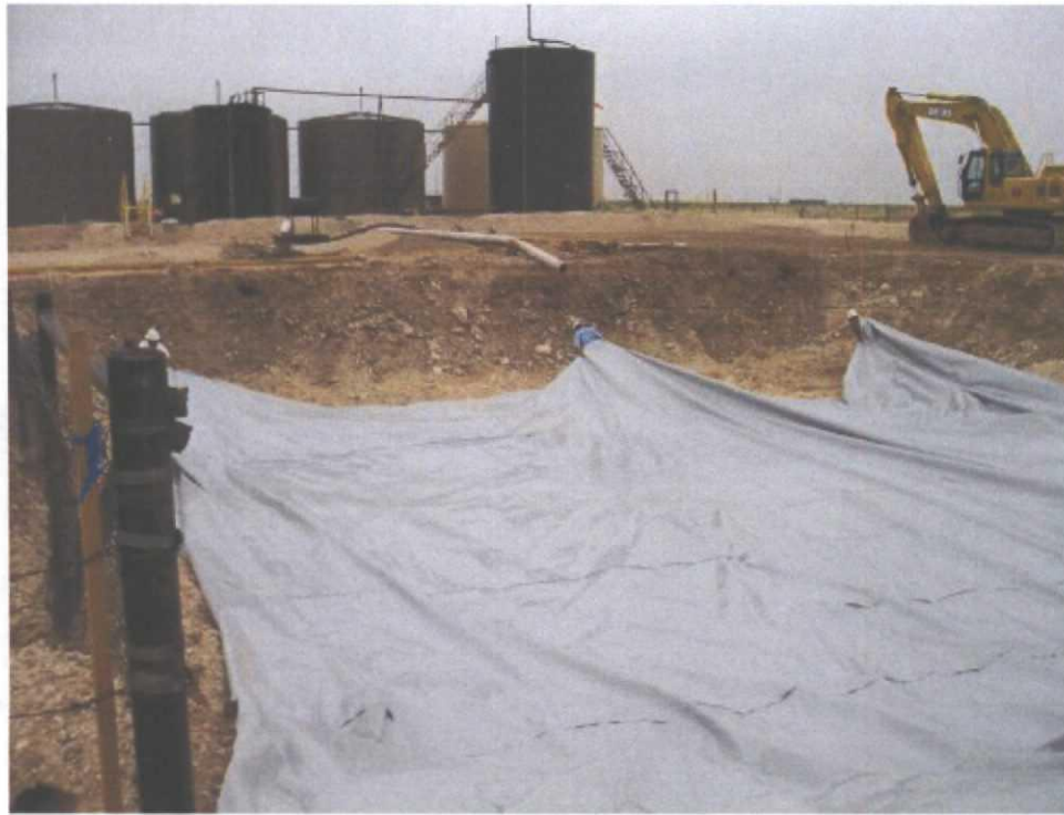
Liner Being Placed into Pit
