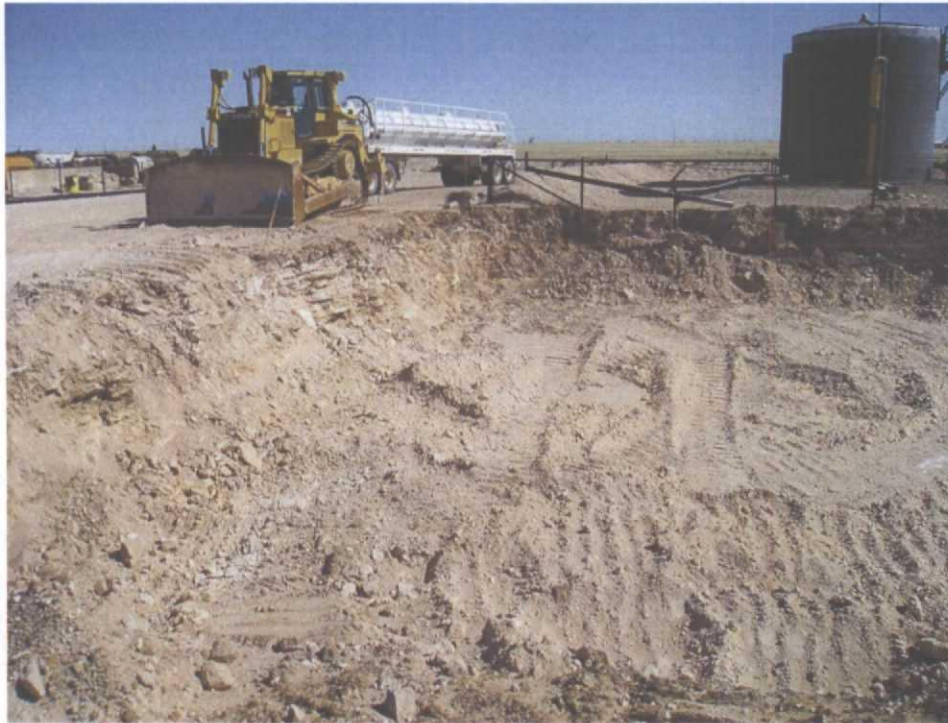
Pit Closure Following Concrete Removal
