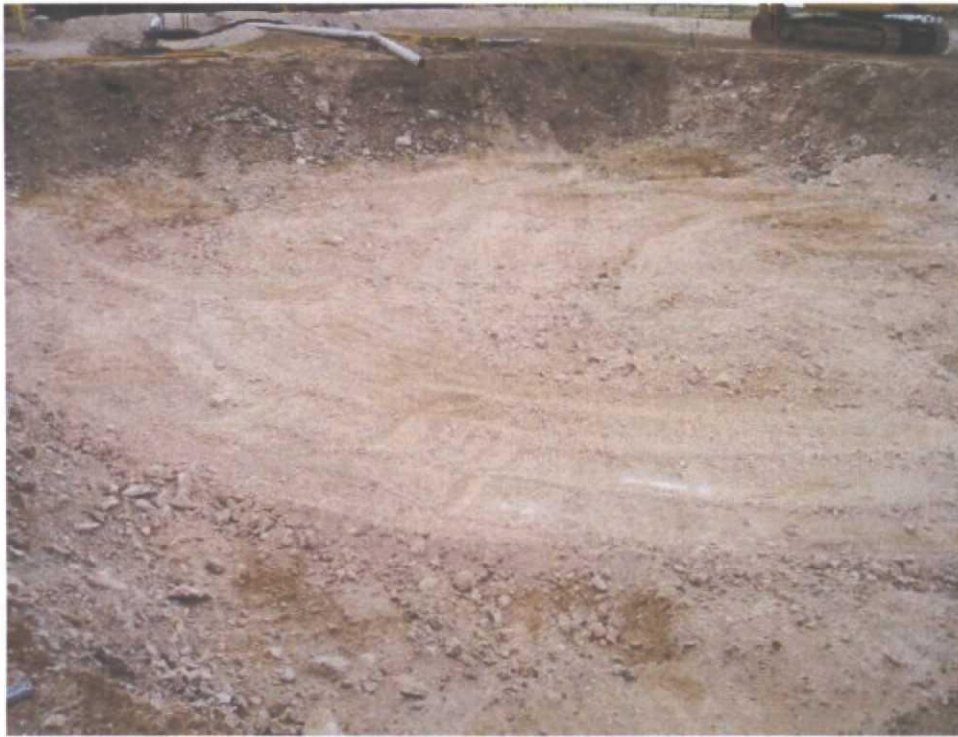
Pit Prepared for Liner Installation
