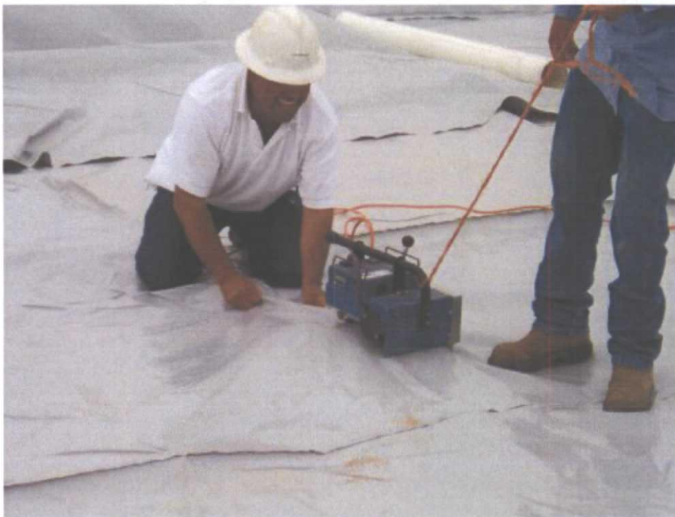
Seaming Liner for Installation
