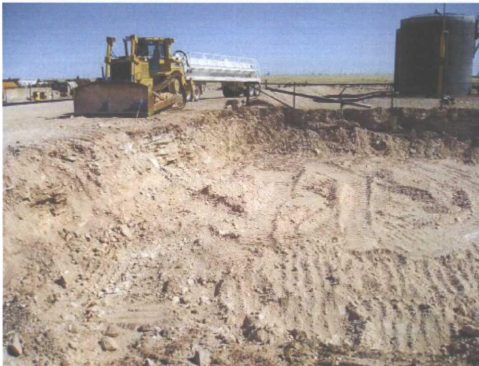
Backfilling Excavation
