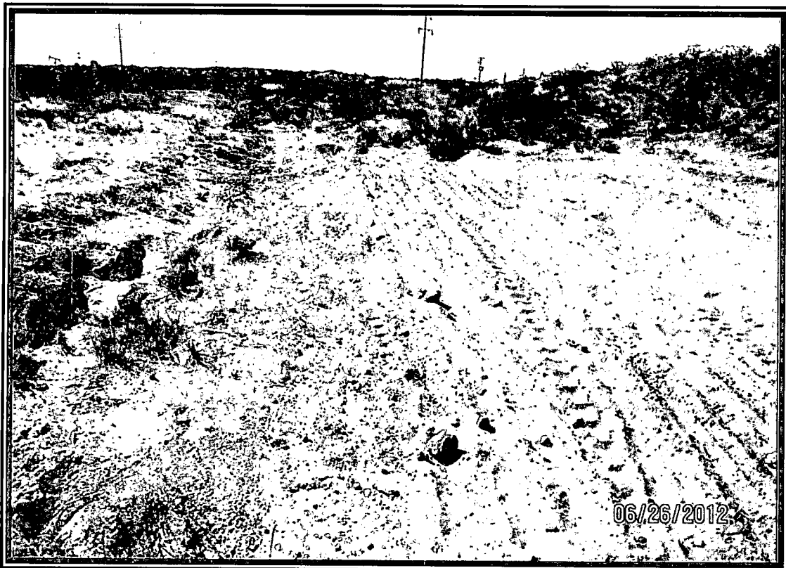
View of spill area after backfill, seeding and water bars were installed.
