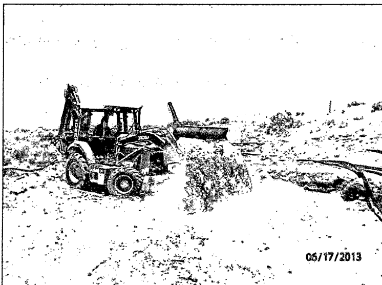
Backfilling the site with clean, imported caliche, facing southwest 6/17/13
