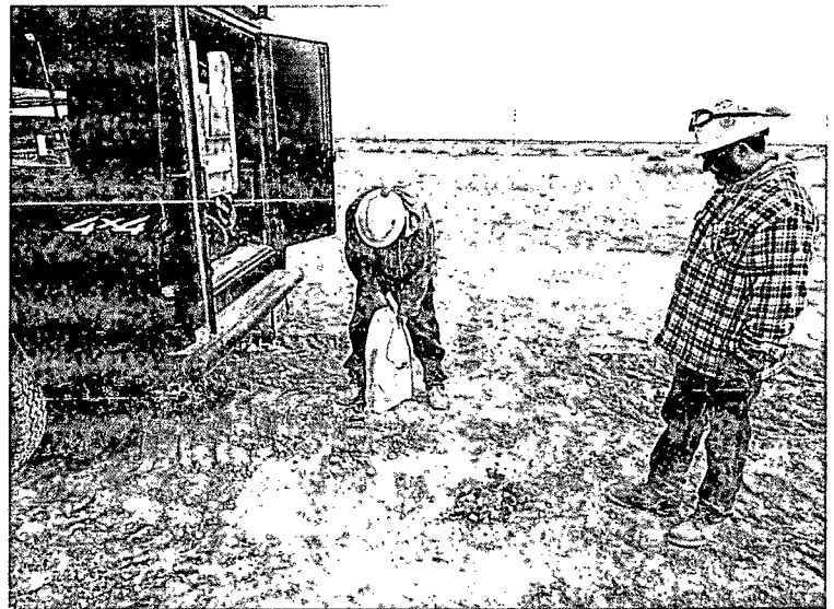
Plugging Pt. 3 bore in total with bentonite
