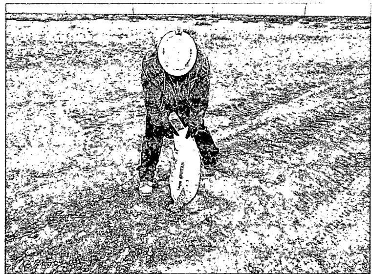
Plugging Pt. 5 bore in total with bentonite
