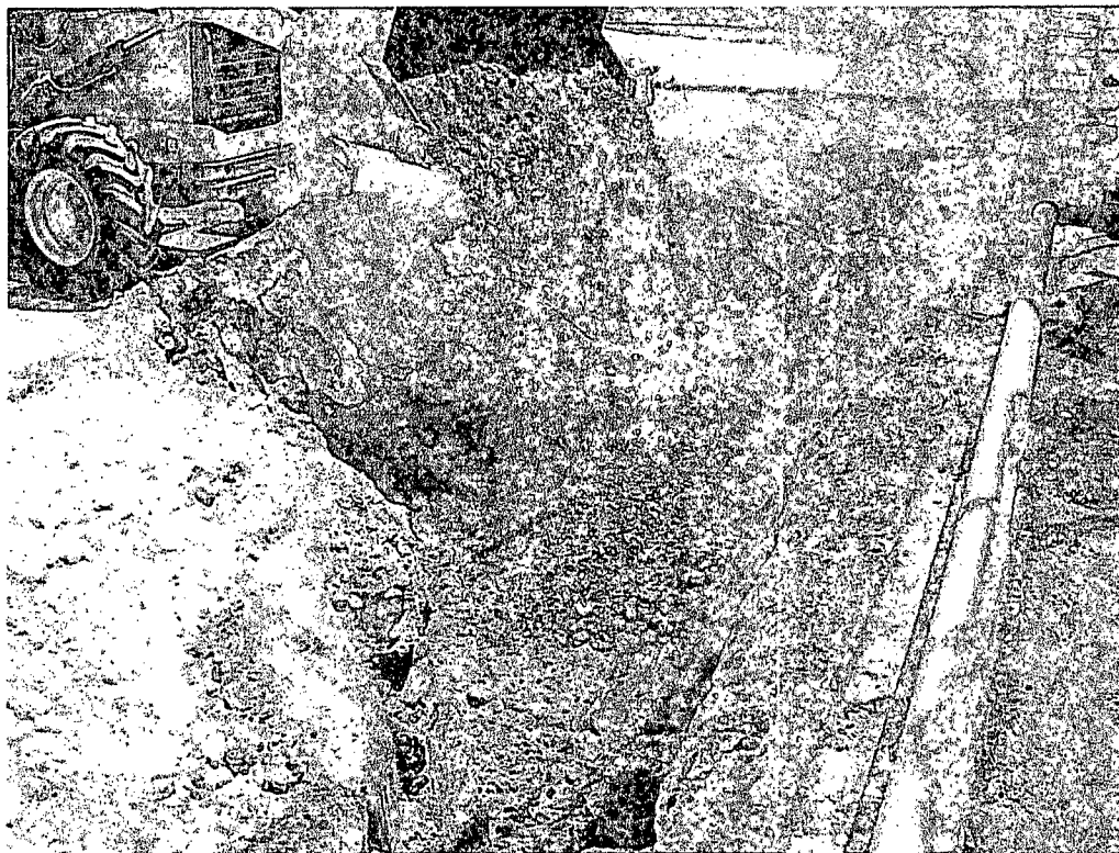
View of excavation clay capping
