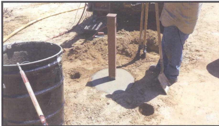
Photo 10: Installation of protective bollards around MW-1.
