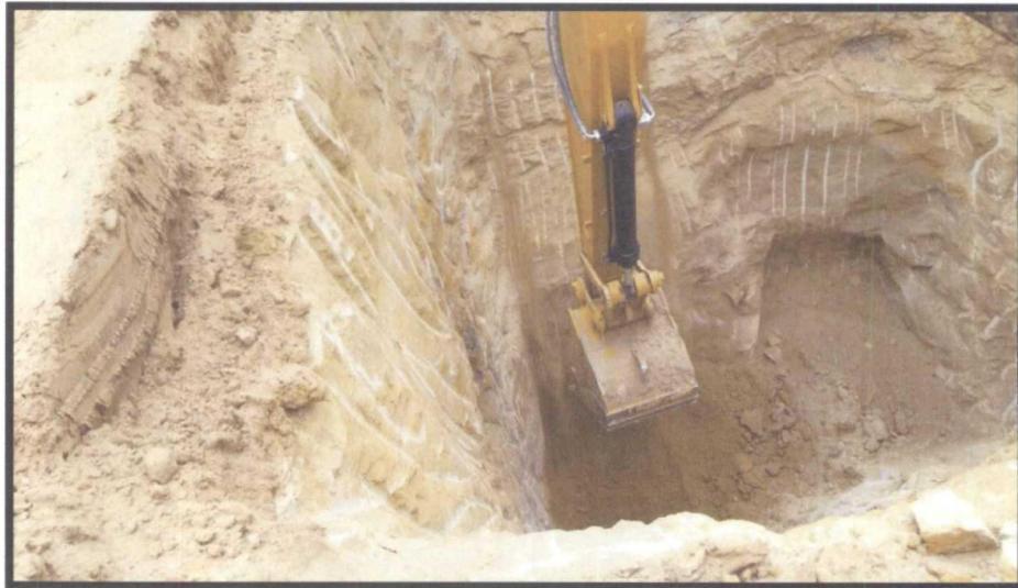
Photo 4: Trunk K #8 at total depth (37' BGS), samples collected as composites from multiple bucket scrapes against sandstone bedrock. Very competent sandstone visible to depth.
