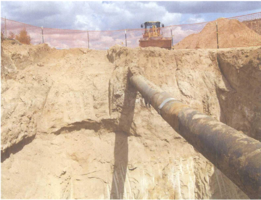
Trench 2 with repaired pipe.
