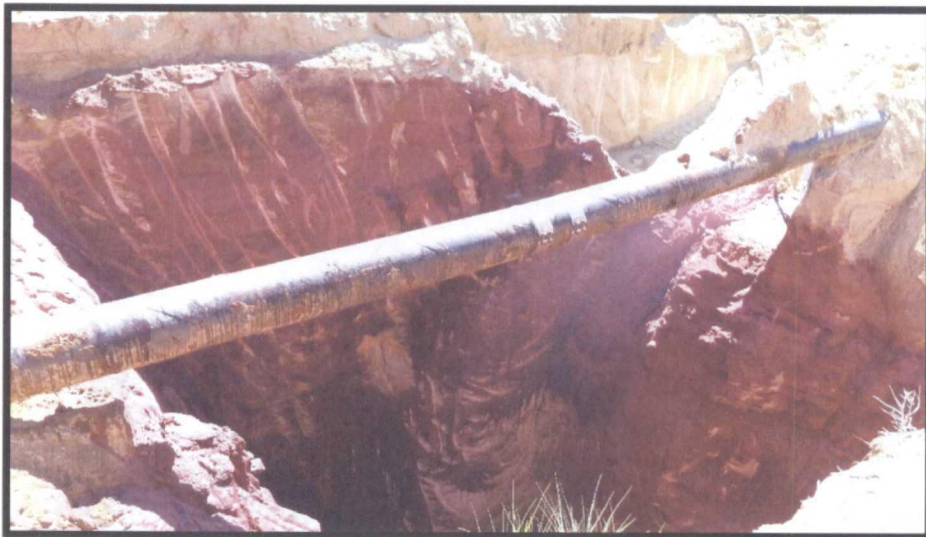
Photo 6: Trunk K #8 excavation after potassium permanganate application.
