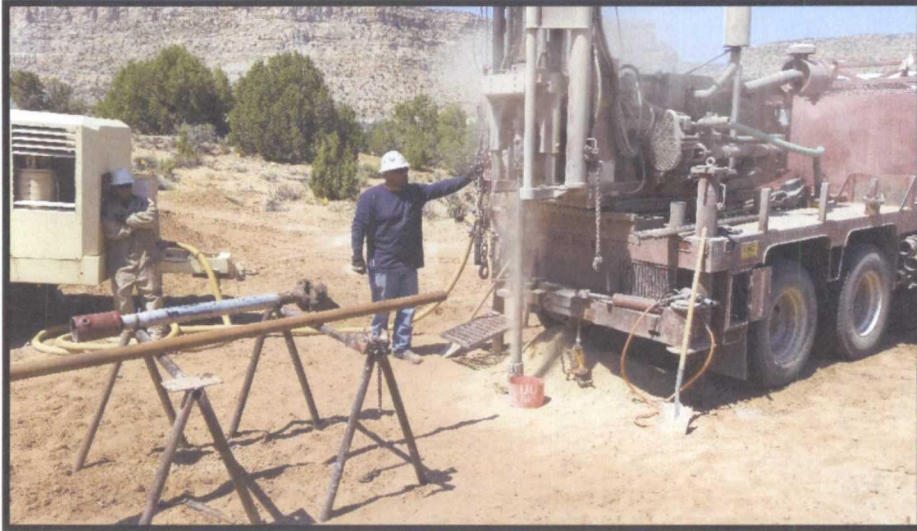
Photo 7: Soil coring drilling method collecting soil samples at the Trunk K #8 release location after potassium permanganate application and backfill.
