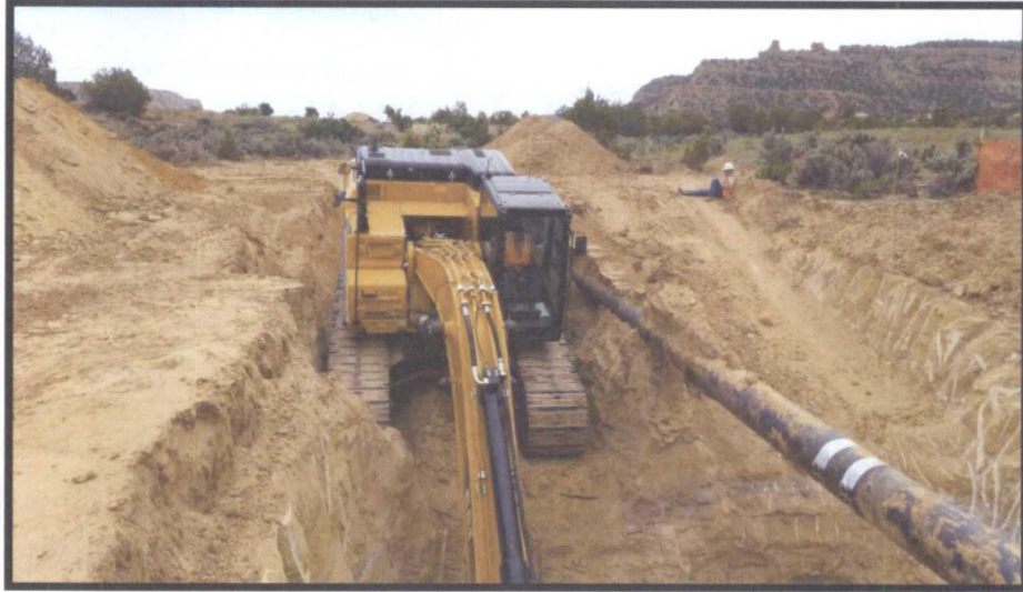
Photo 3: Trunk K #8 Final depth measured 37' BGS. Photo shows deepest bench on NE side of excavation.
