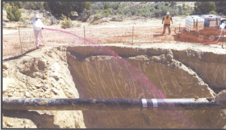
Photo 5: Potassium Permanganate application at the Trunk K #8 excavation.
