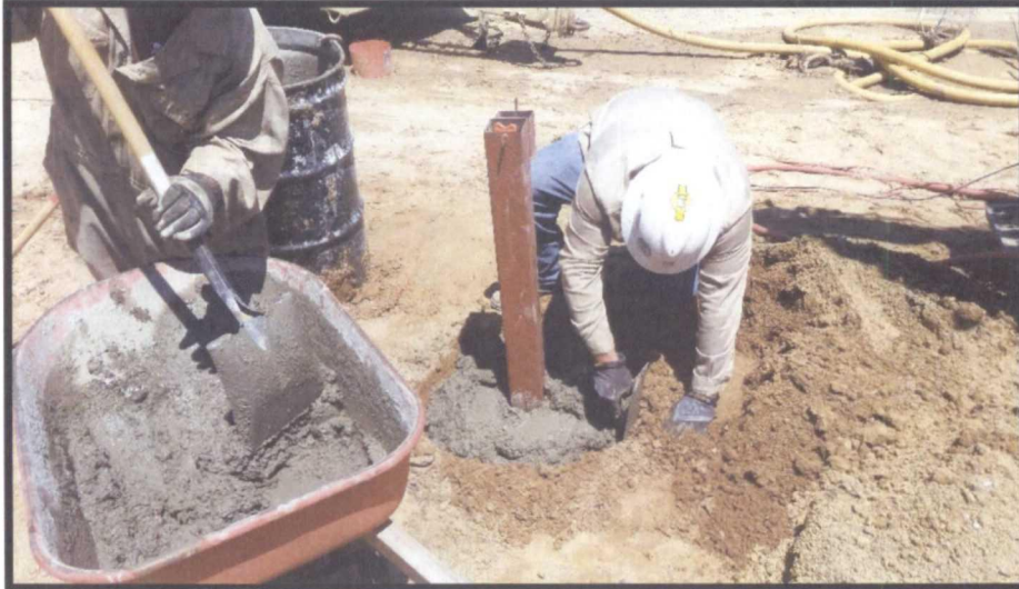
Photo 9: Installation of above ground protective well cover for MW-1.
