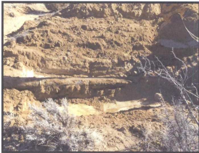
Photo 2: Trunk K #8 excavation encountered competent sandstone at a shallow depth, the sandstone unit extended to below the total depth of the excavation.
