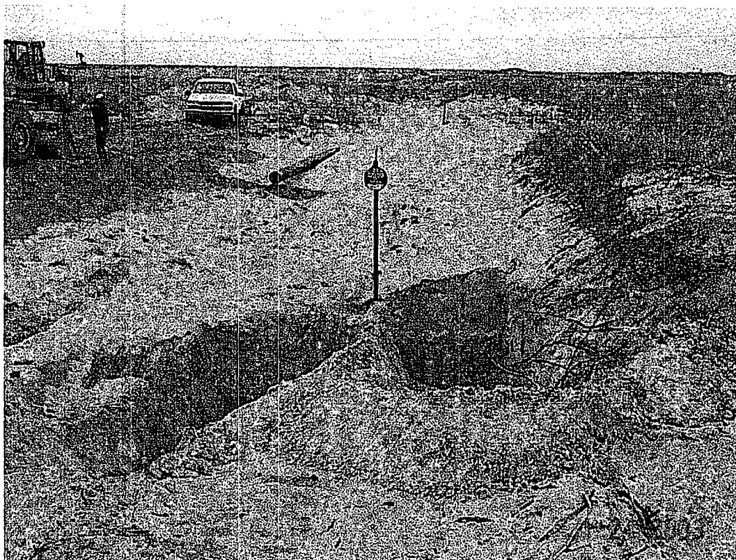
1 View facing west showing initial excavation. Pipeline marker (center) marks where 12-inch steel line (west side) is joined with 10-inch poly line (east side) along active pipeline. Inactive 12-inch steel pipeline (upper left) is shown where a 200-ft section was cut off and removed. 01-24-03
