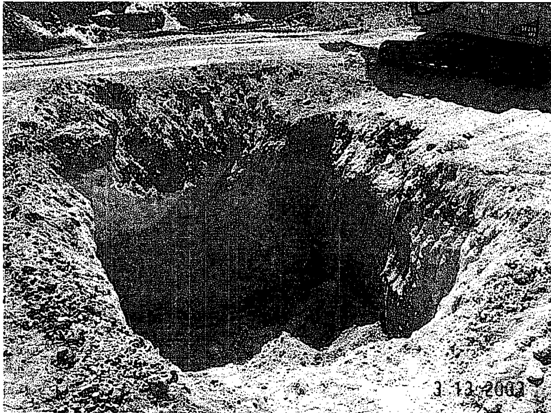
6 View facing southwest showing floor (20 ft below surface) and the south and west walls at completion of excavation activities.
