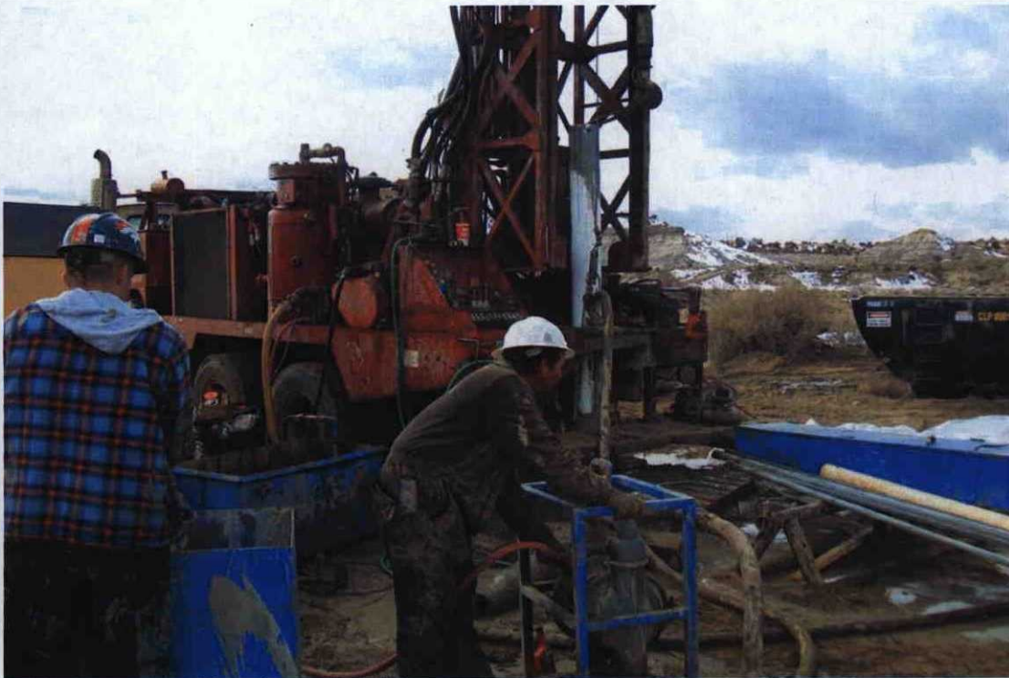
Photo 3: View of drilling surface casing cementing operations.
