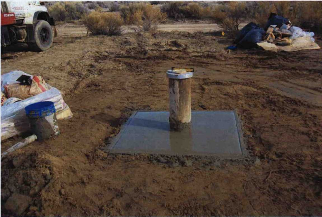
Photo 9: View of surface completion for MW-1.
