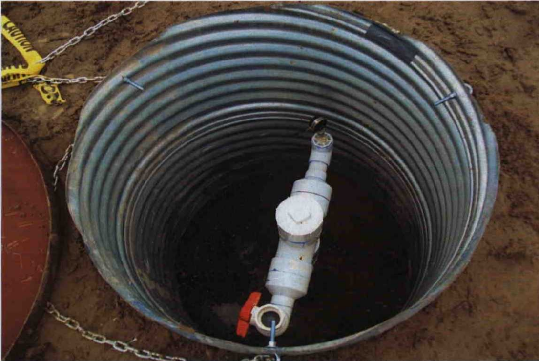
Photo 10: View of of the below grade well head completion for MW-2.
