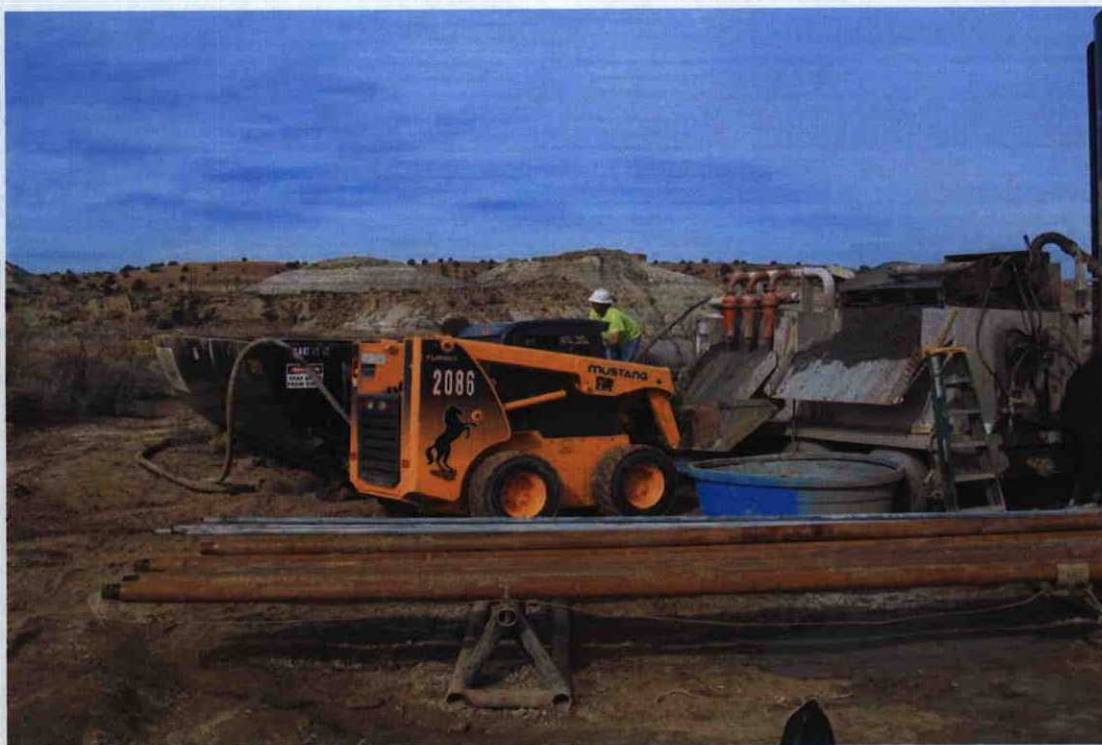
Photo 5: View of mud tank and cuttings shaker.
