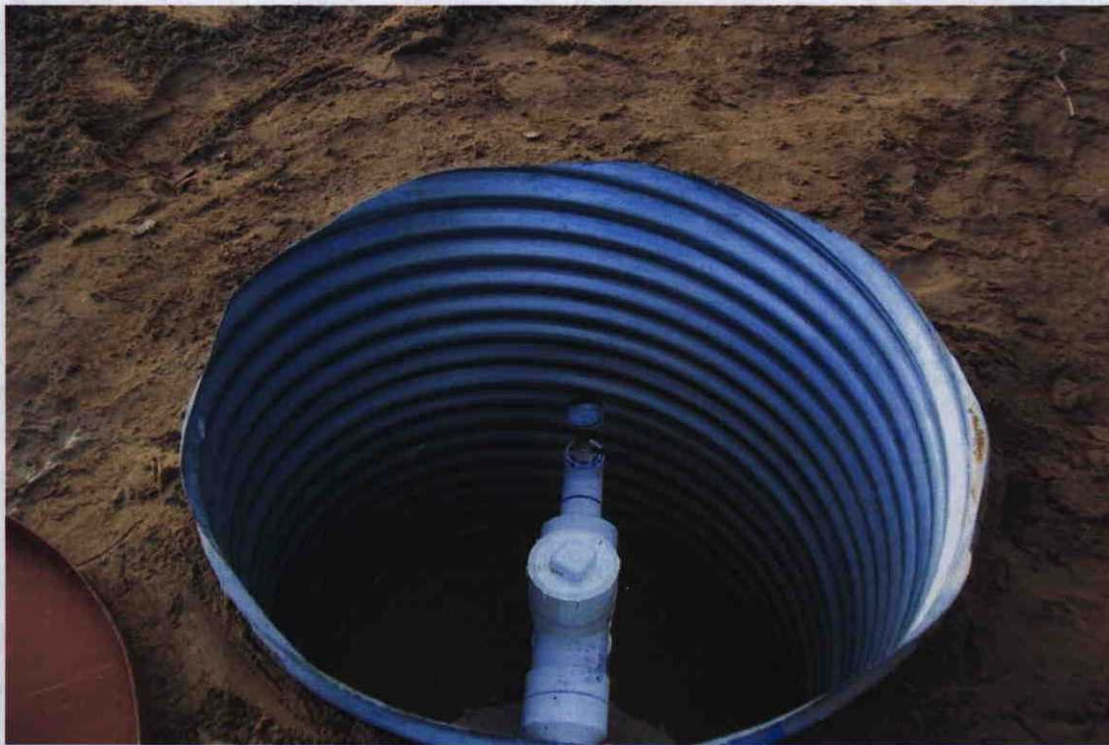
Photo 11: View of the below grade well head completion for MW-3.
