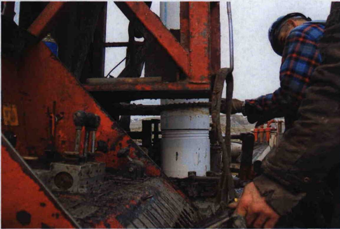
Photo 2: View of surface casing installation.
