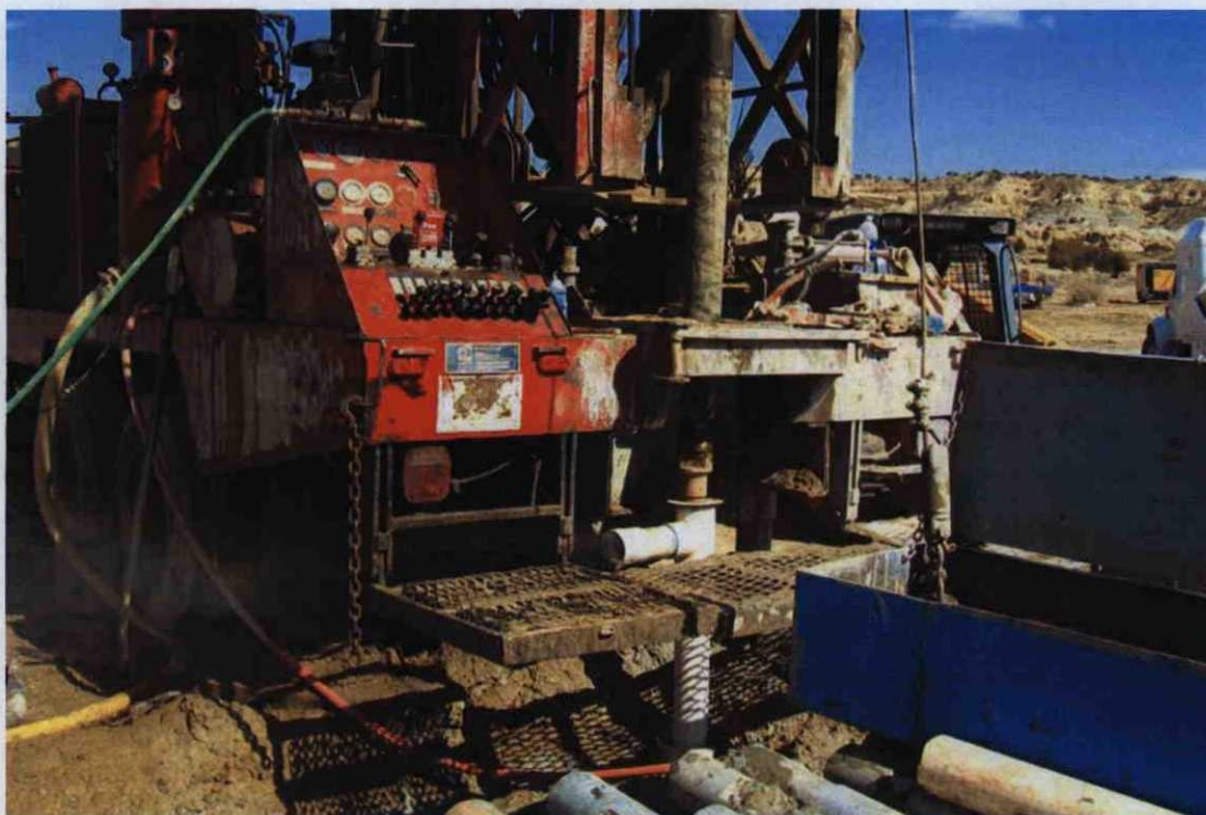
Photo 8: View of the air lifting well development.
