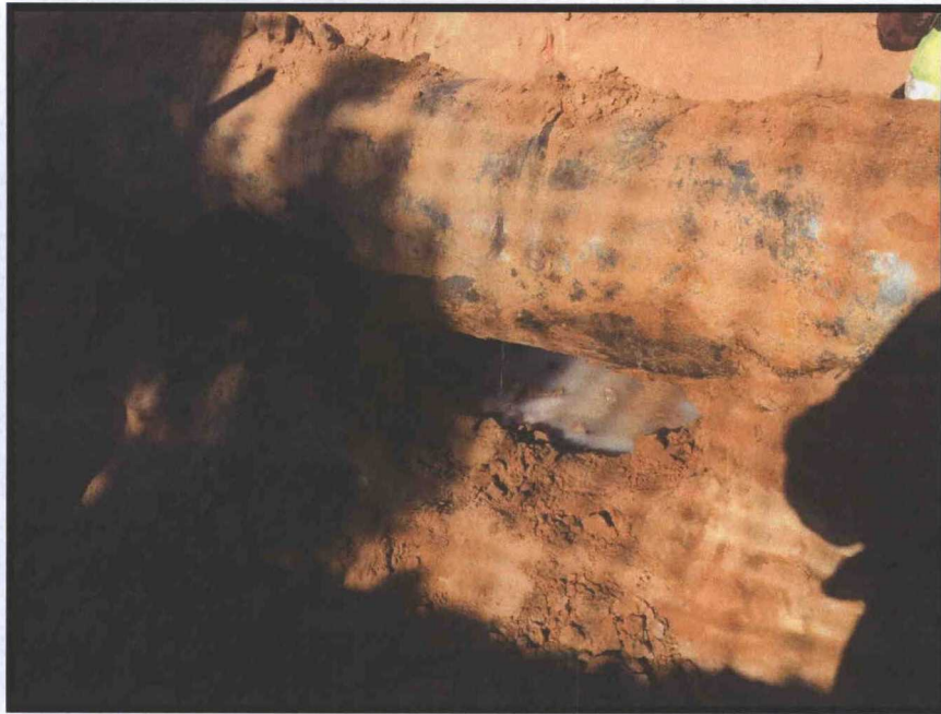
Photo 1: Trunk K #9 Excavation exposes the release point.
