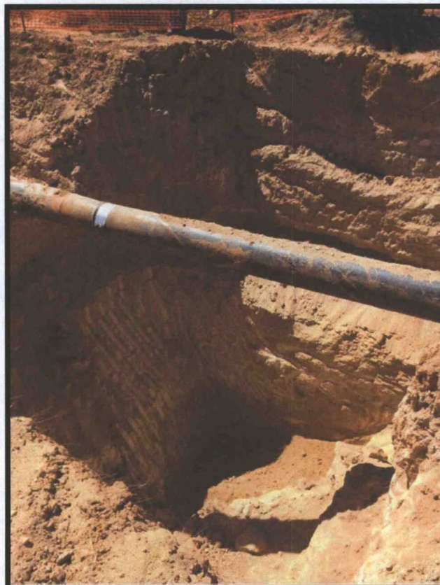
Photo 3: Trunk K #9 Excavation encountered Sandstone at about 7 feet BGS.
