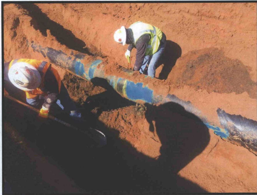
Photo 1: Trunk K #5 Excavation showing failed I-wrap repairs, impacted soil being removed from beneath the pipeline.
