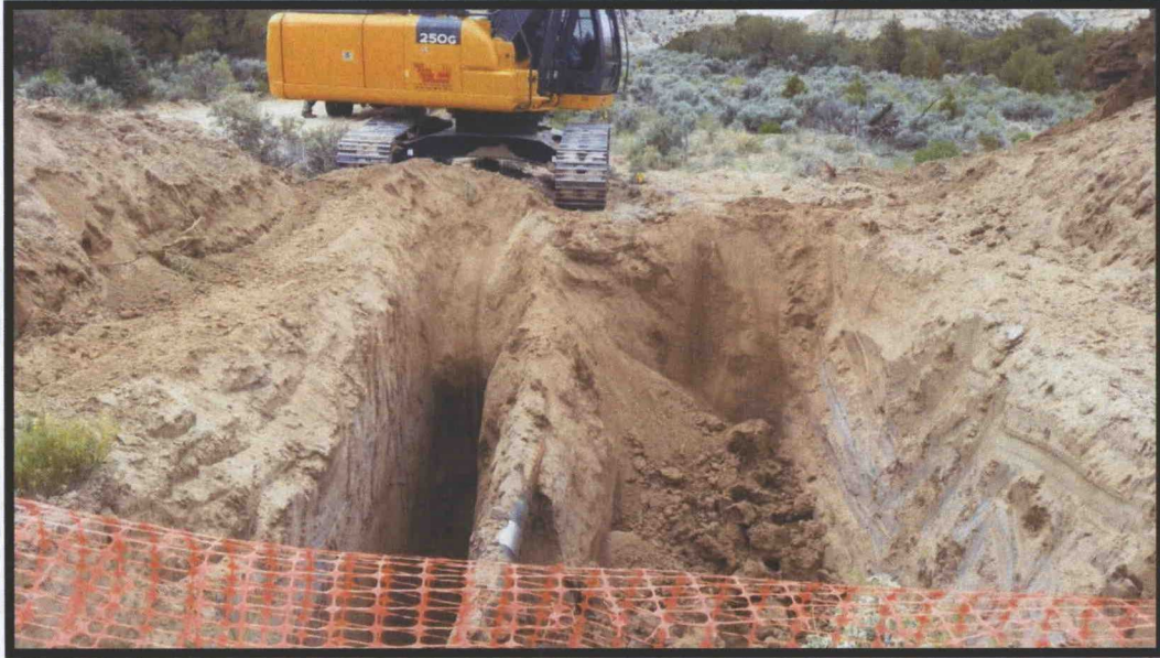
Photo 3: Lateral 2A-4 South excavation at largest extent, loose material on north side (right) of excavation was removed shortly after this photo.
