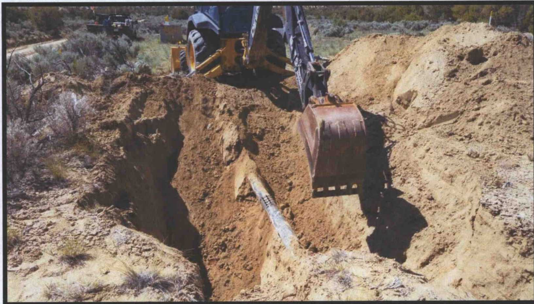
Photo 2: Excavation with rubber tire backhoe after clamp was installed. The excavation quickly became too large for the equipment on site and a track mounted excavator was scheduled for the following day.
