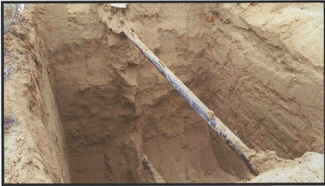
Photo 3: Lateral 2A-4 North excavation at largest extent, soil consisted of loose, fine to medium grained sands, with little to no coherence.
