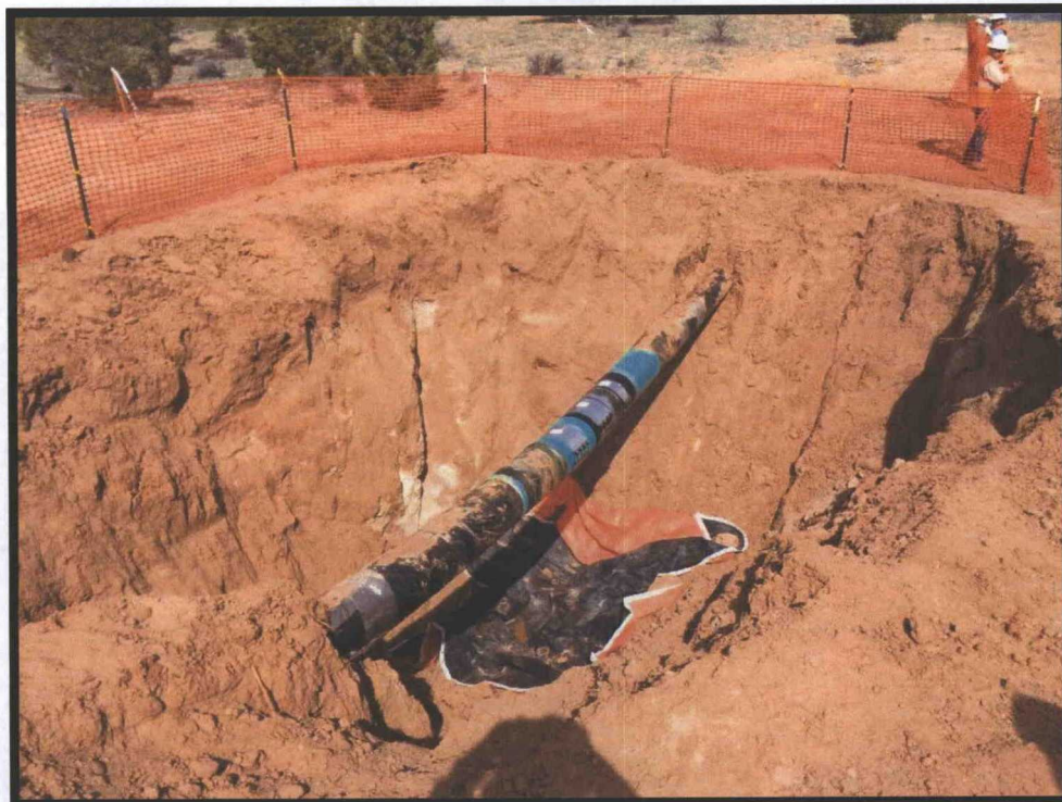
Photo 3: Trunk K #6 Excavation waiting for repair, plastic liner used to catch any liquids dripping from pipe before repairs took place.
