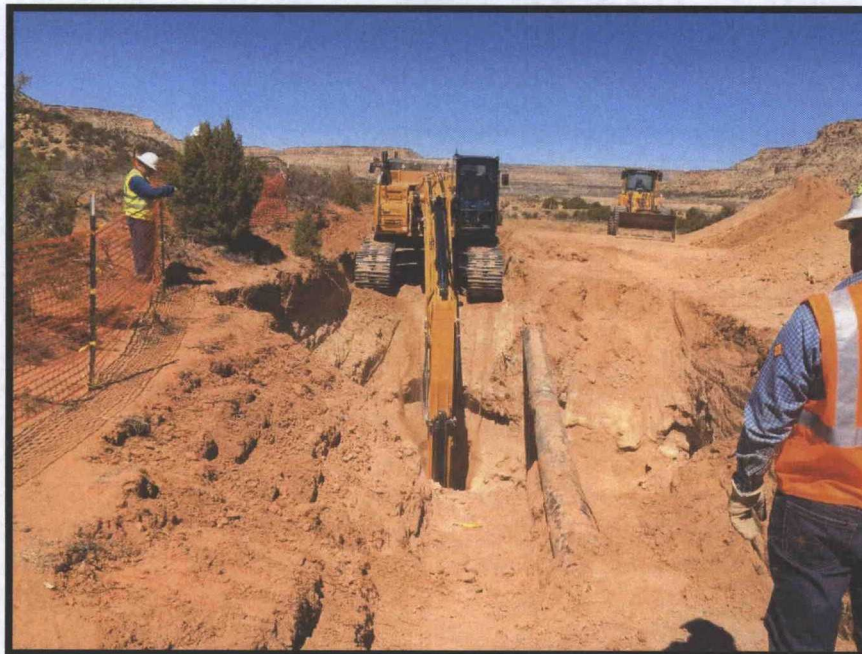
Photo 2: Trunk K #9 Excavation increasing in depth through sandstone.
