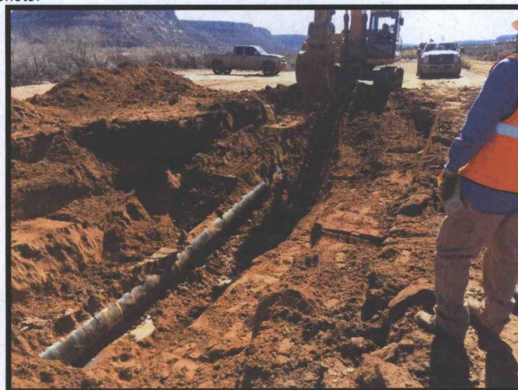
Photo 1: Trunk K #2 release point, result of failed I-Wrap repair, liquids visible in photo.
