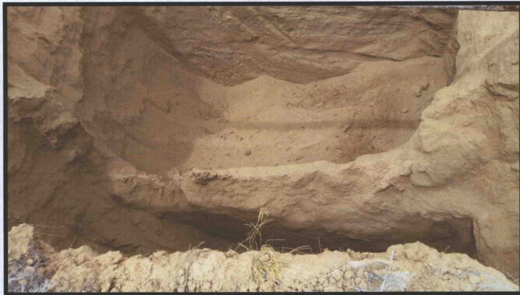
Photo 4: Excavation base at maximum depth of 20' BGS after sampling activities, loose material visible is result of collecting sidewall samples. Base sample was collected first.
