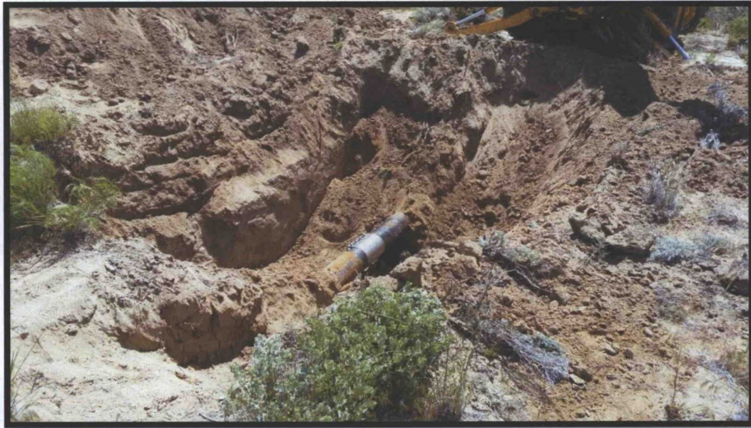
Photo 1: Lateral 2A-4 South site, initial excavation for pipeline inspection and repair, photo aspect to south west. Soil material consists of tight dry sandy clay.
