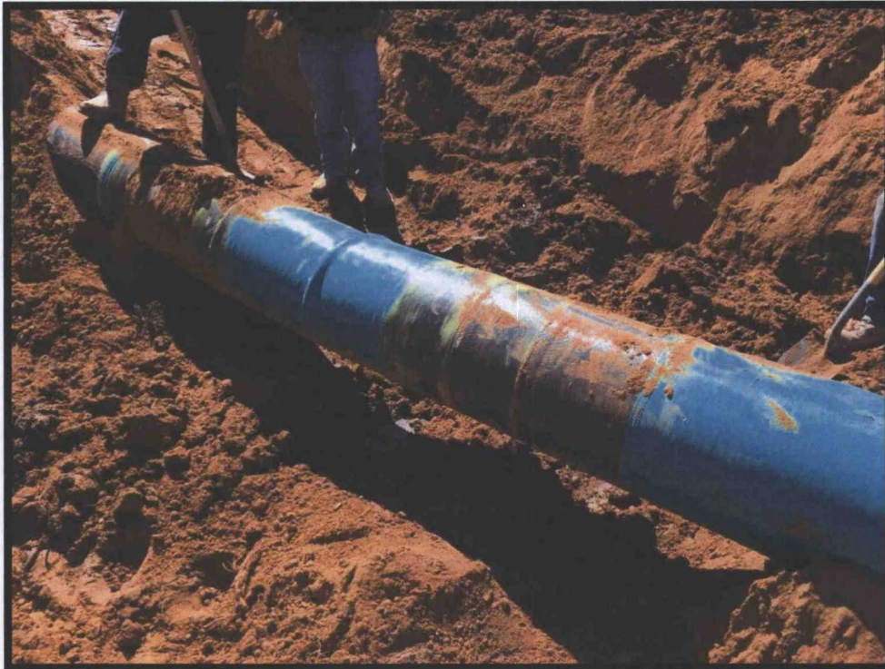
Photo 1: Trunk K #6 Excavation exposes the failed I-Wrap repair from October 2014.
