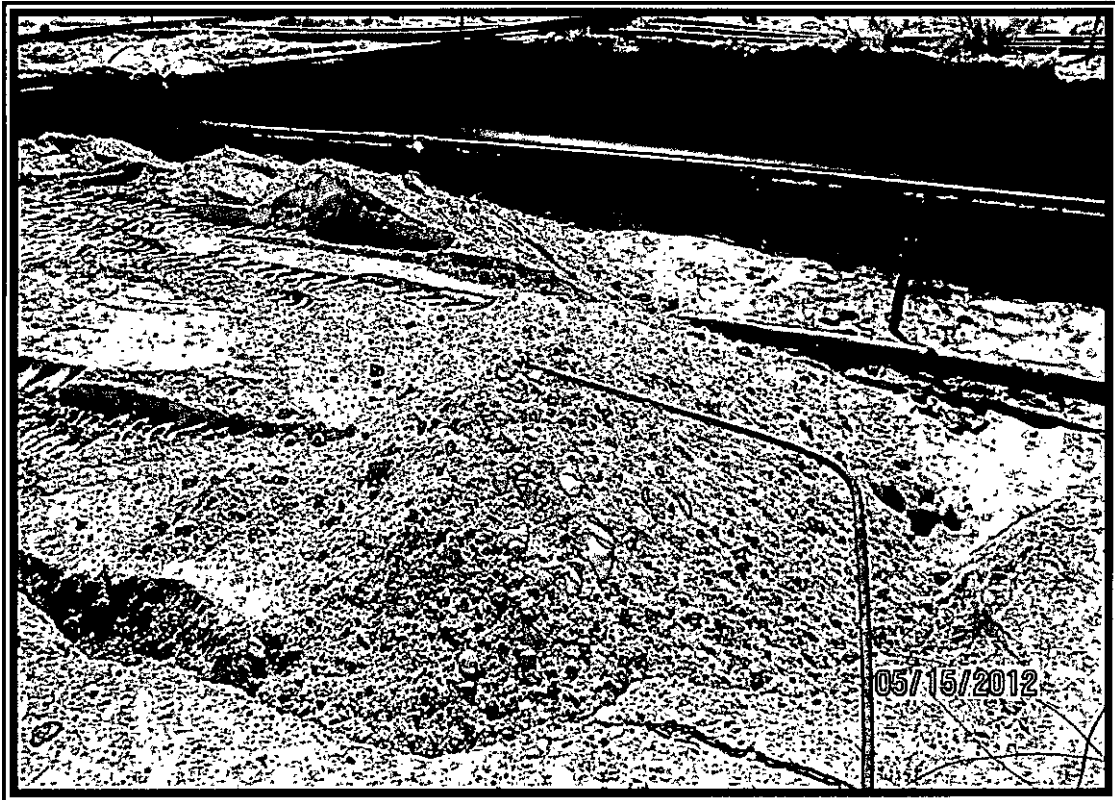
View of the excavation after gypsum was put in place during the backfill.
