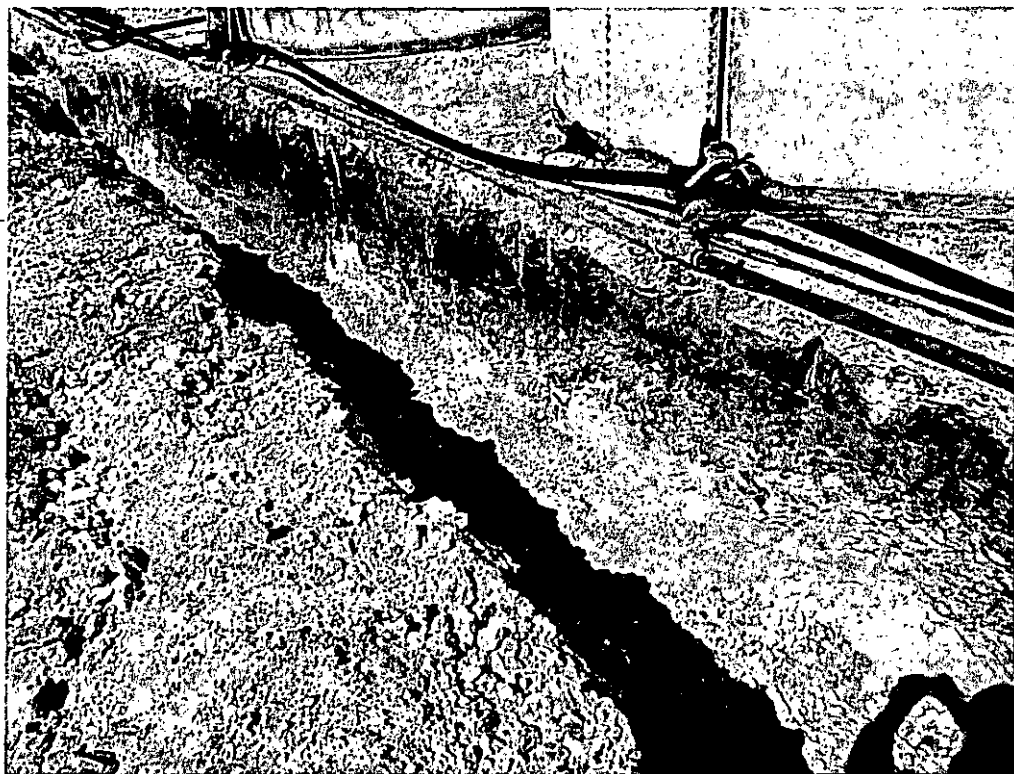
View Northwest – Area of AH-2
