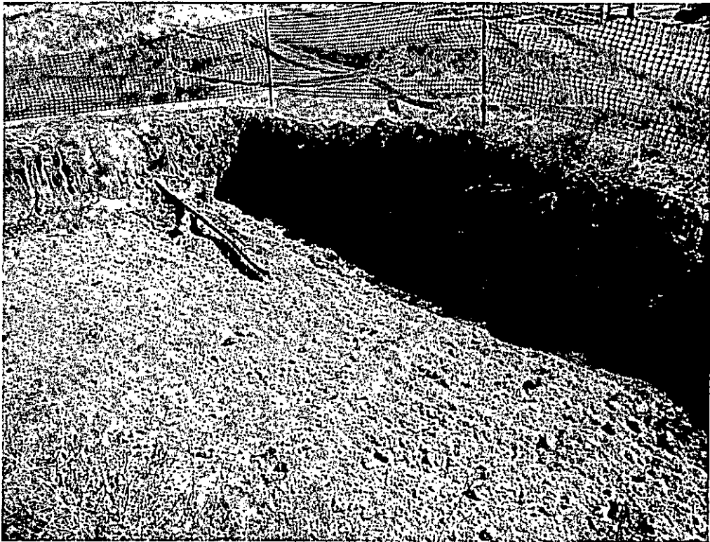
Final depth of excavation from 4.5' to 5.5'
