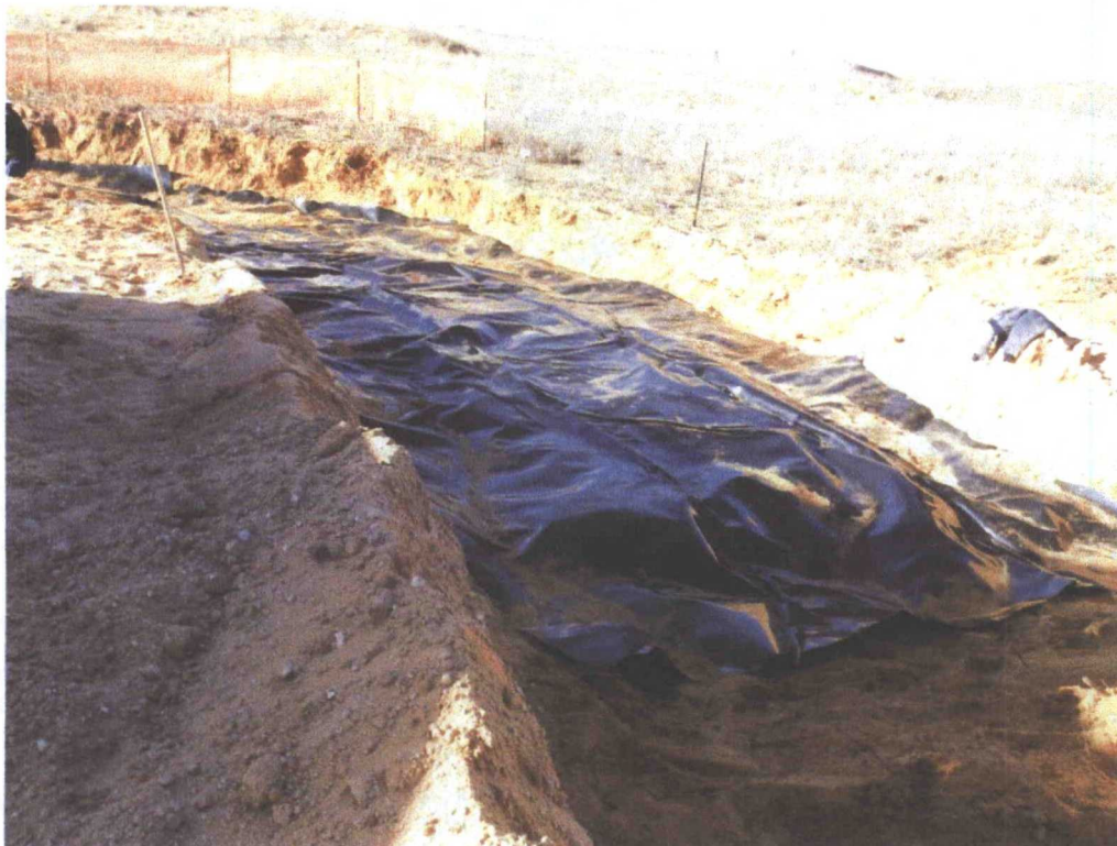
View South - Liner
