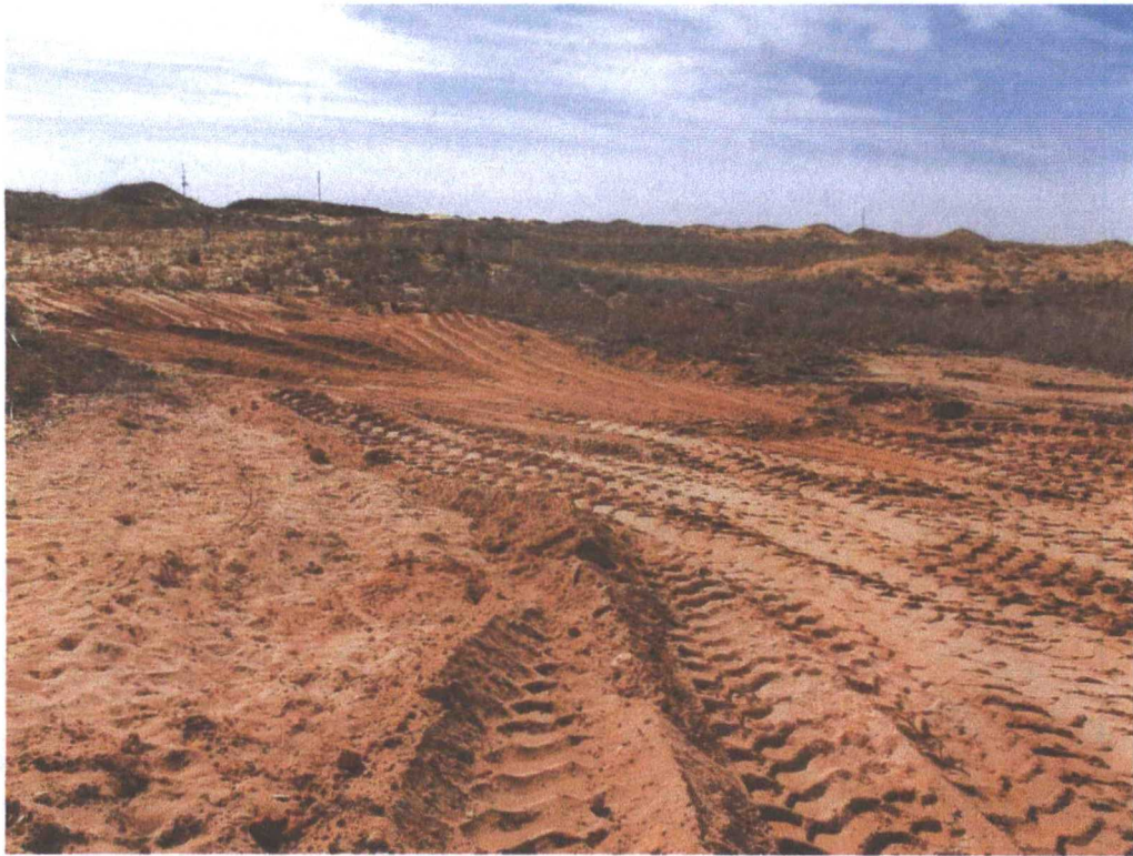
View South – Backfill and Rip
