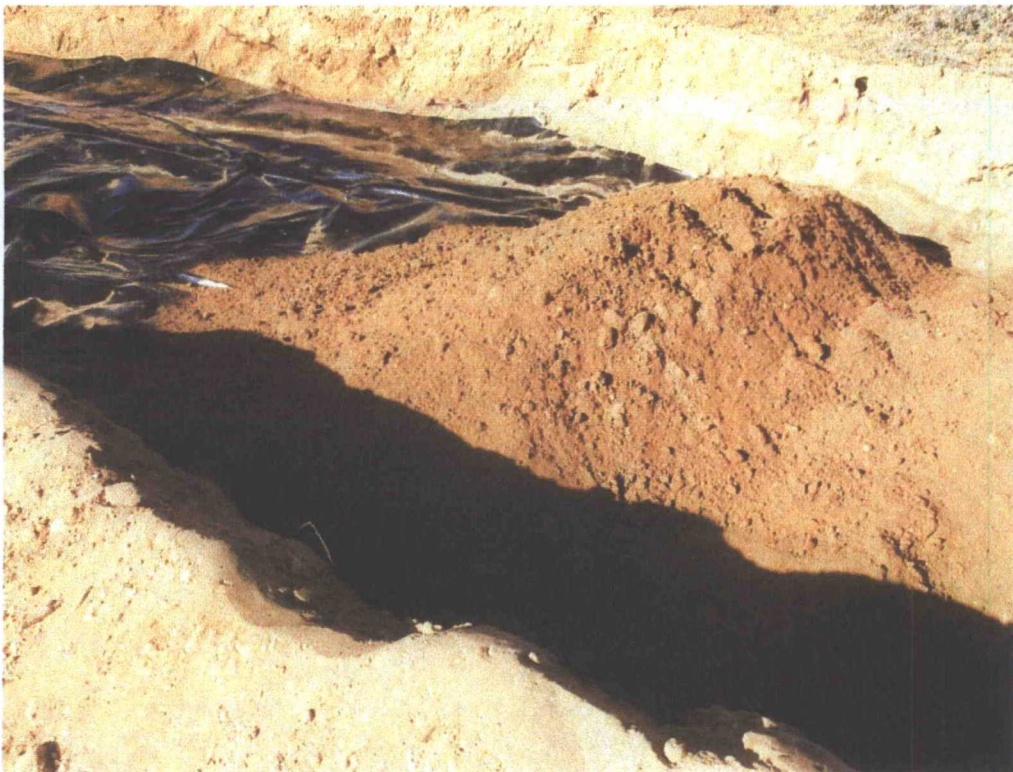
View Southwest - Backfill
