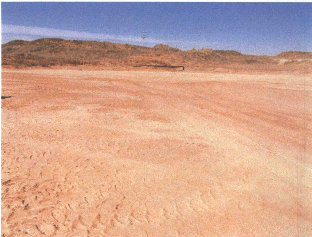
View West - Backfill
