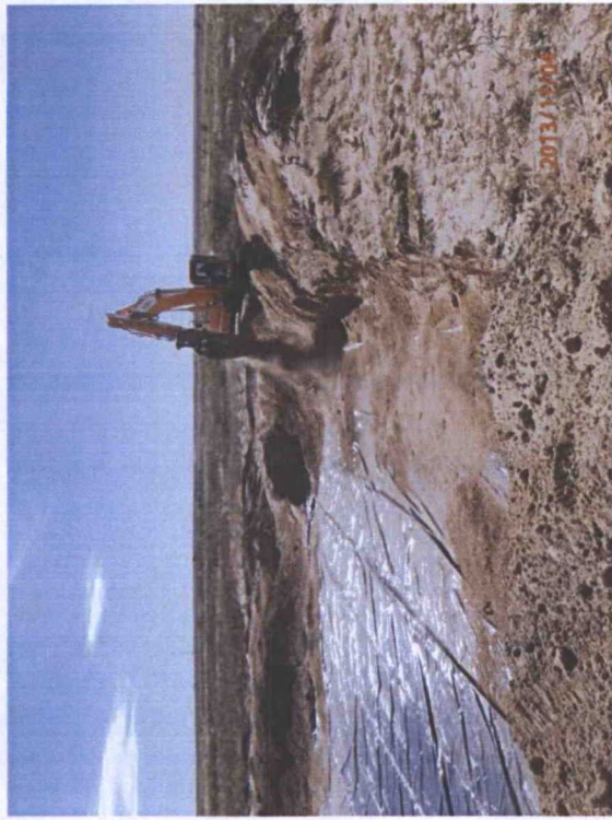
Backfilling over liner, facing south 11/4/13
