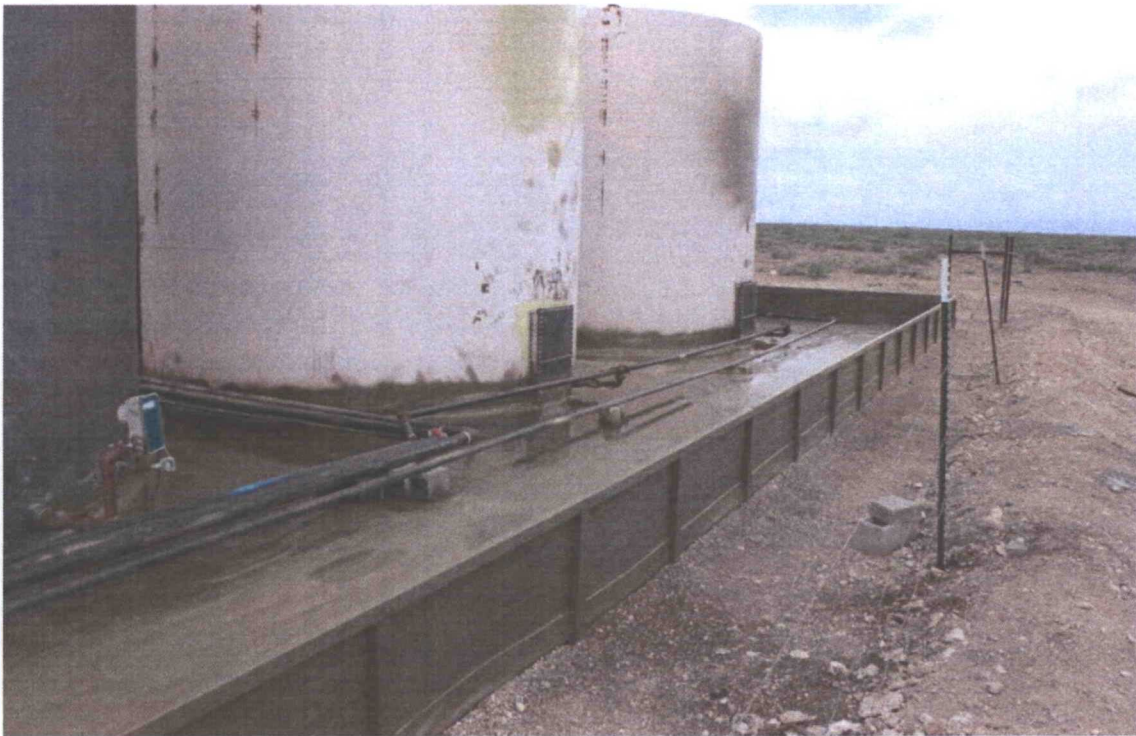
Hat Mesa State 31-32 Battery - Following Liner Installation (looking southeast)
