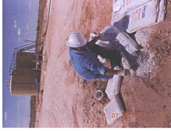
Plugging MW in total with bentonite 7/28/2011
