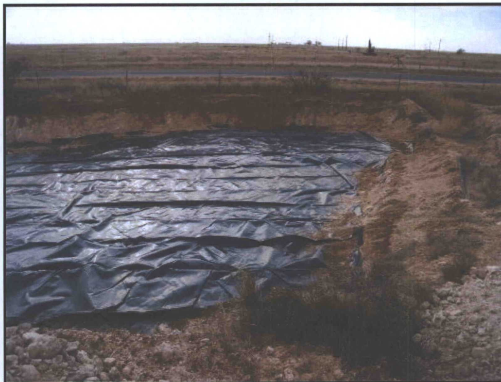
Excavated area lined facing west
