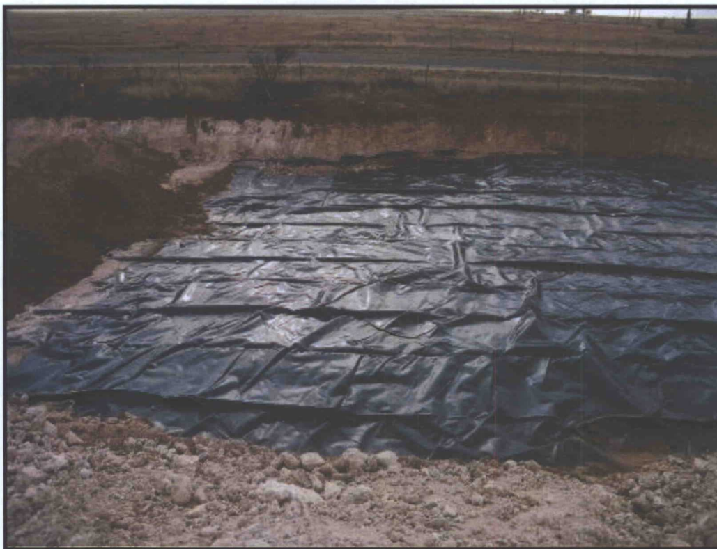
Excavated area lined facing south
