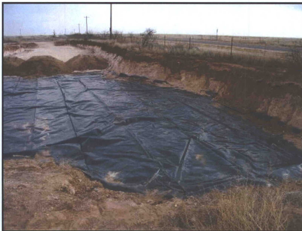
Excavated area lined facing east
