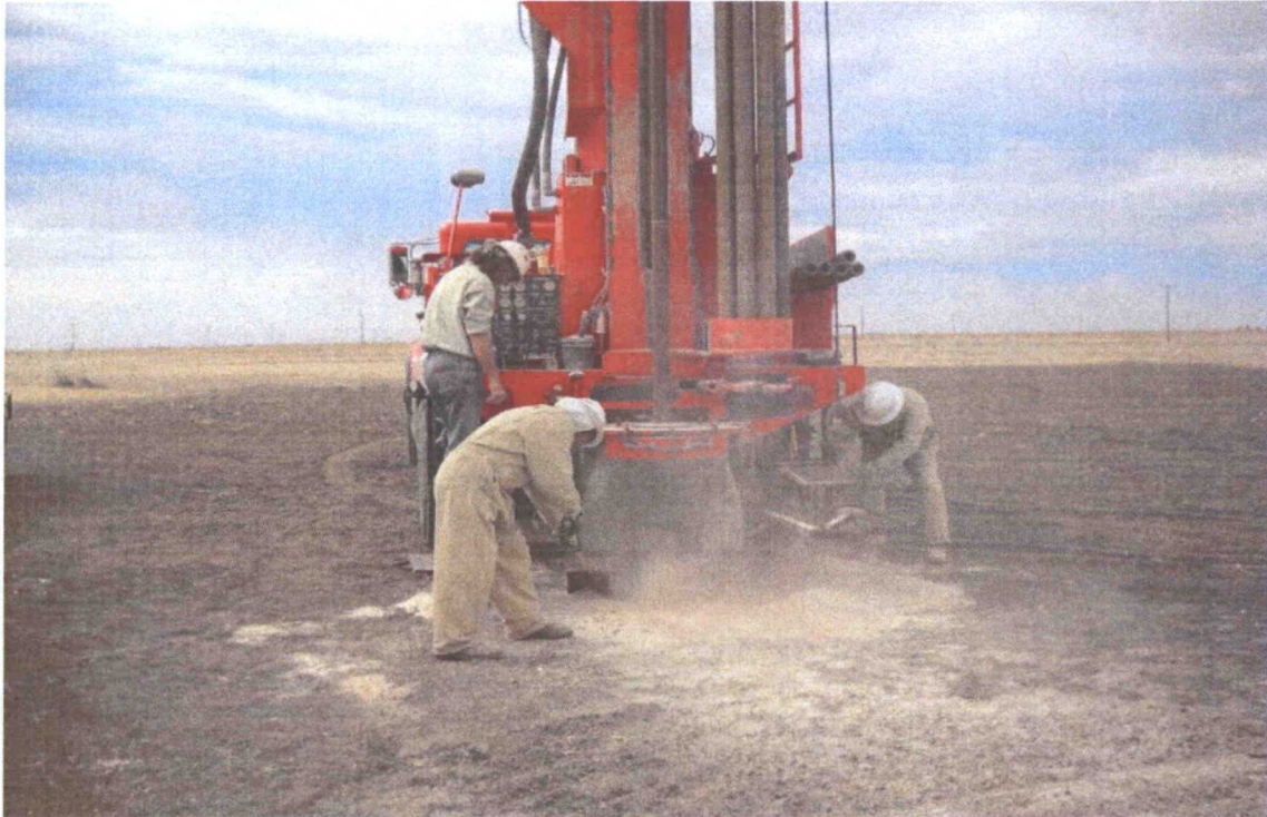
WA Simpson - Advancement of Soil Boring SB-1
