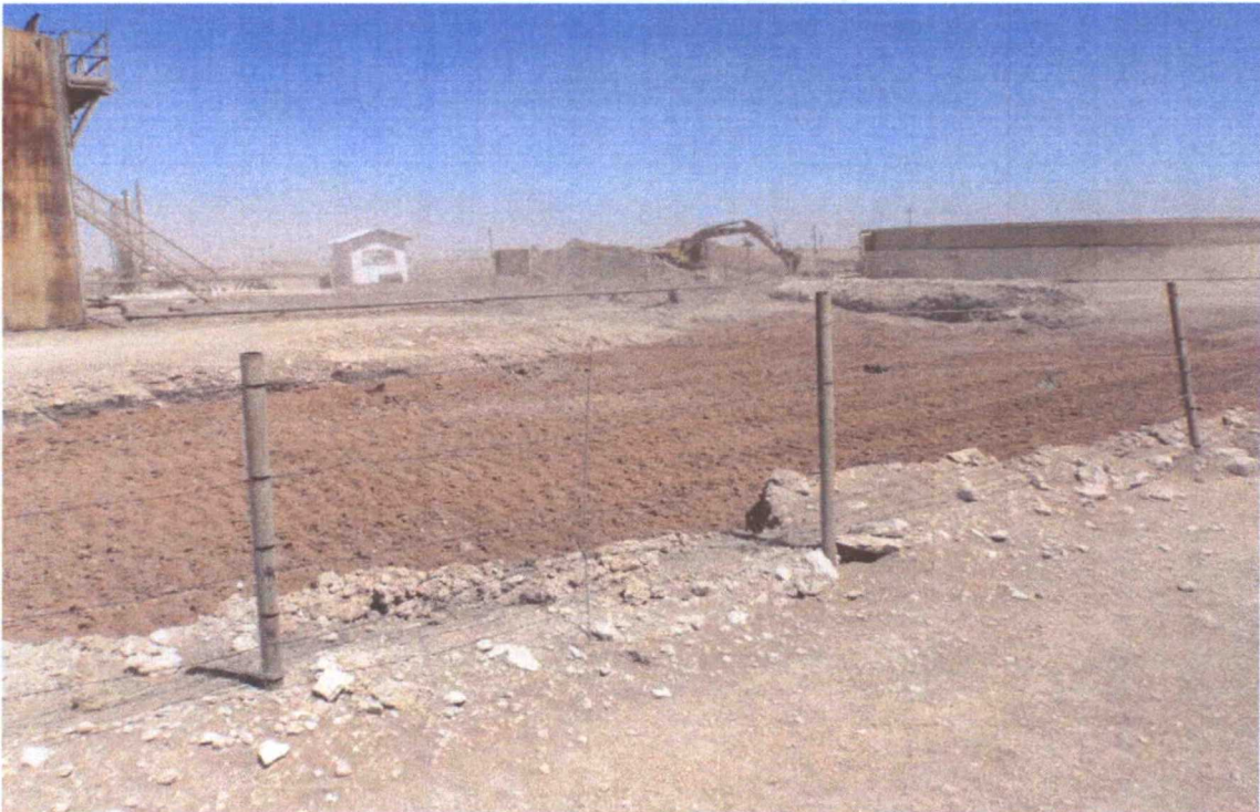
WA Simpson - Tank Battery Excavation (following installation of clay liner)
