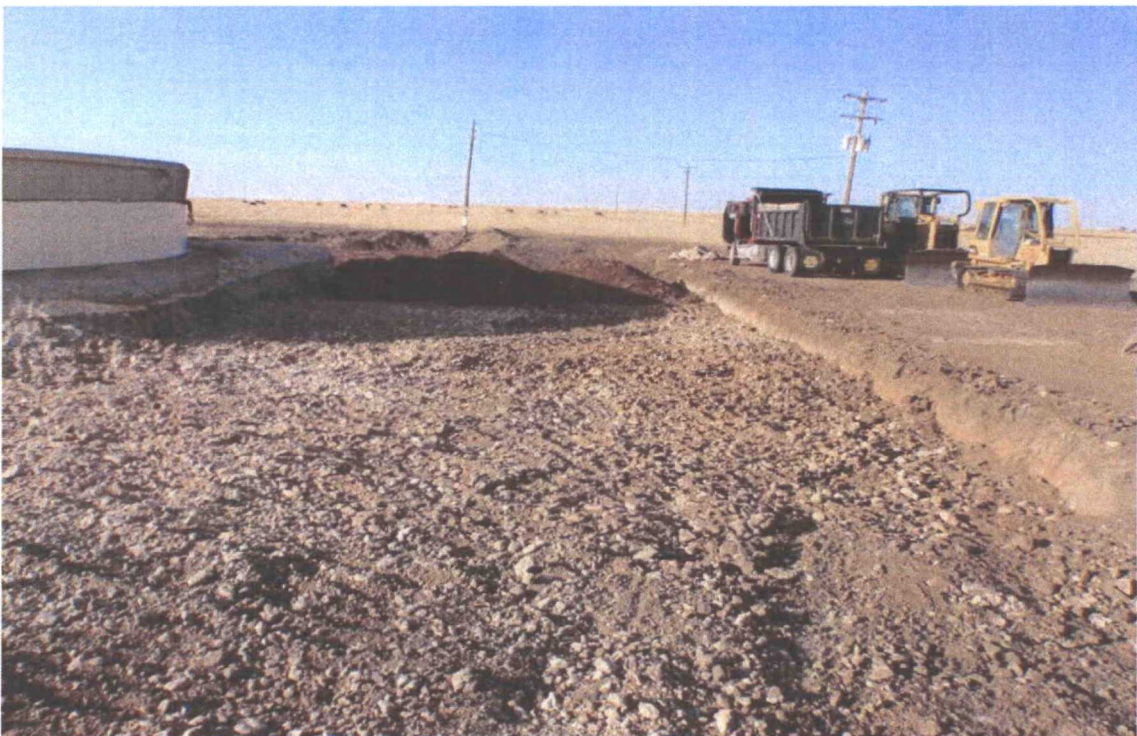
WA Simpson - West Pooling Area Excavation (prior to installation of clay liner; looking west)
