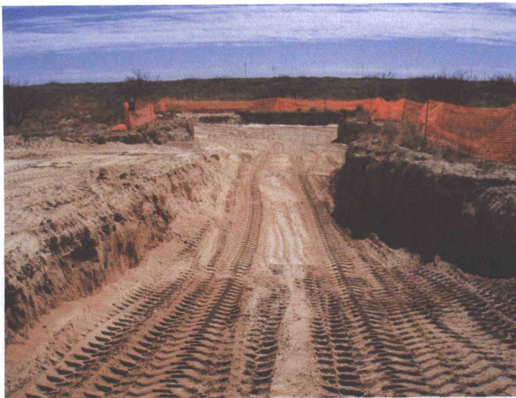
Post excavation – Backfilled to 4' for liner (Along road)
