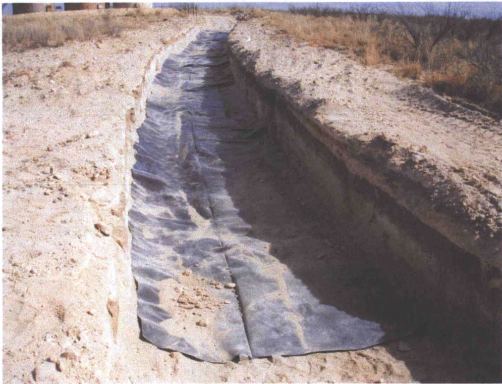
Liner installed along lease road
