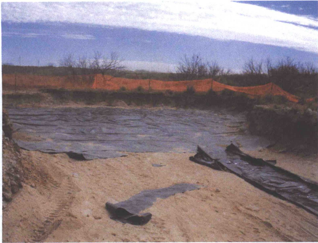
Liner installed in pasture area
