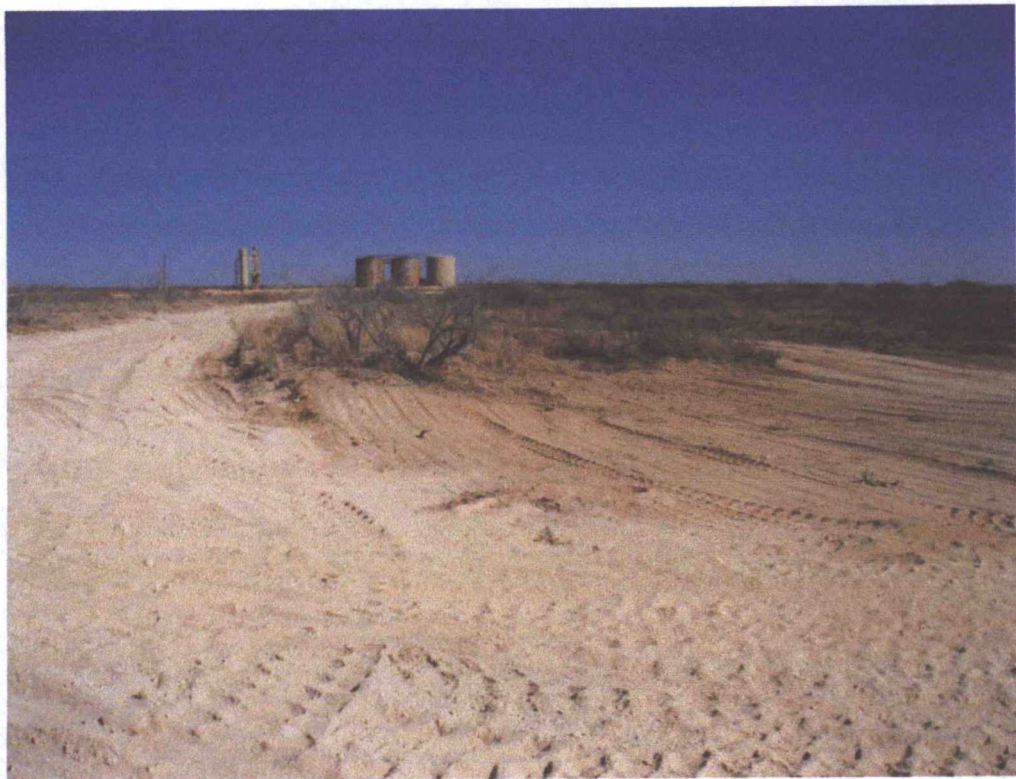
Post remediation and pasture backfilled to surface grade
