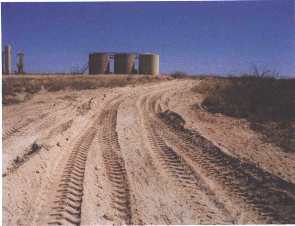
Post remediation and road backfilled to surface grade
