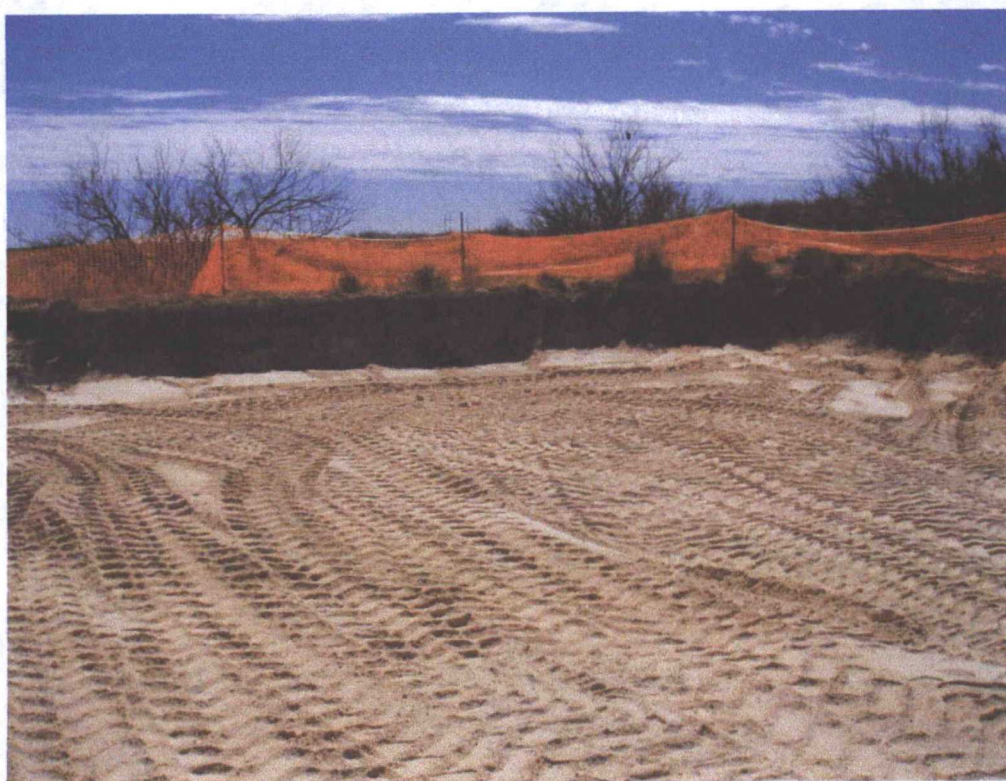
Post excavation – Backfilled to 4' for liner (Pasture area)
