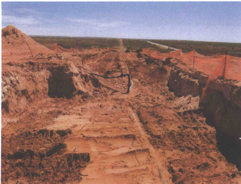
View of Excavation
