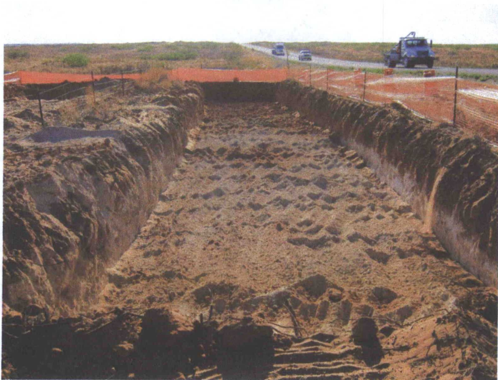
View of Excavation
