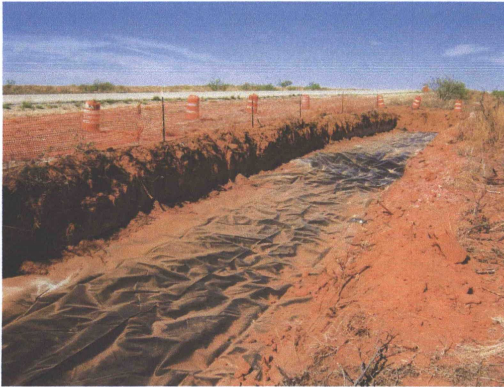
View of Excavation and Liner Installation
