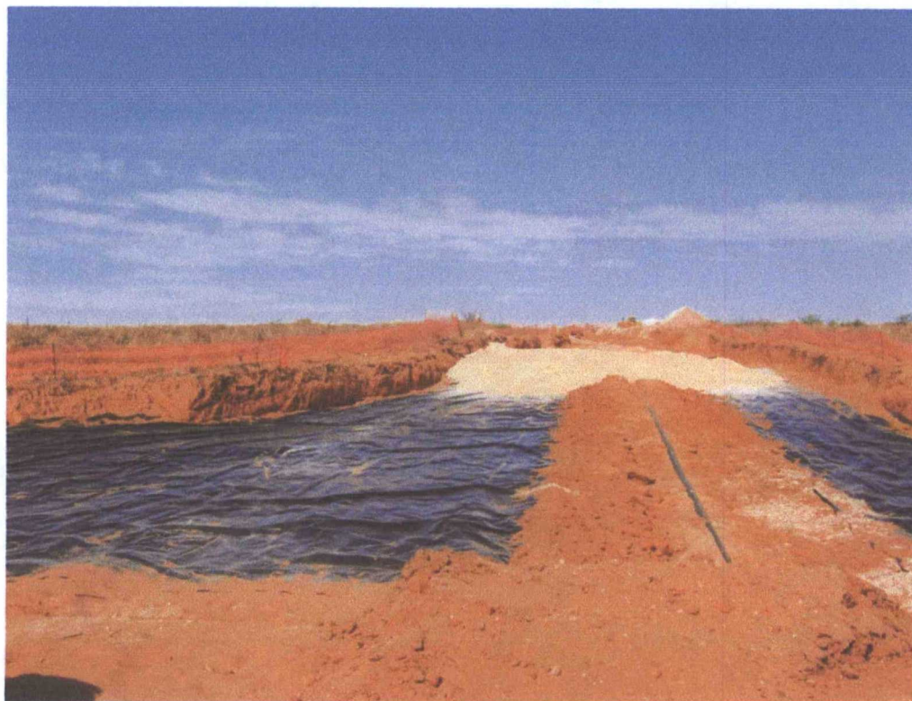
View of Excavation and Liner Installation
