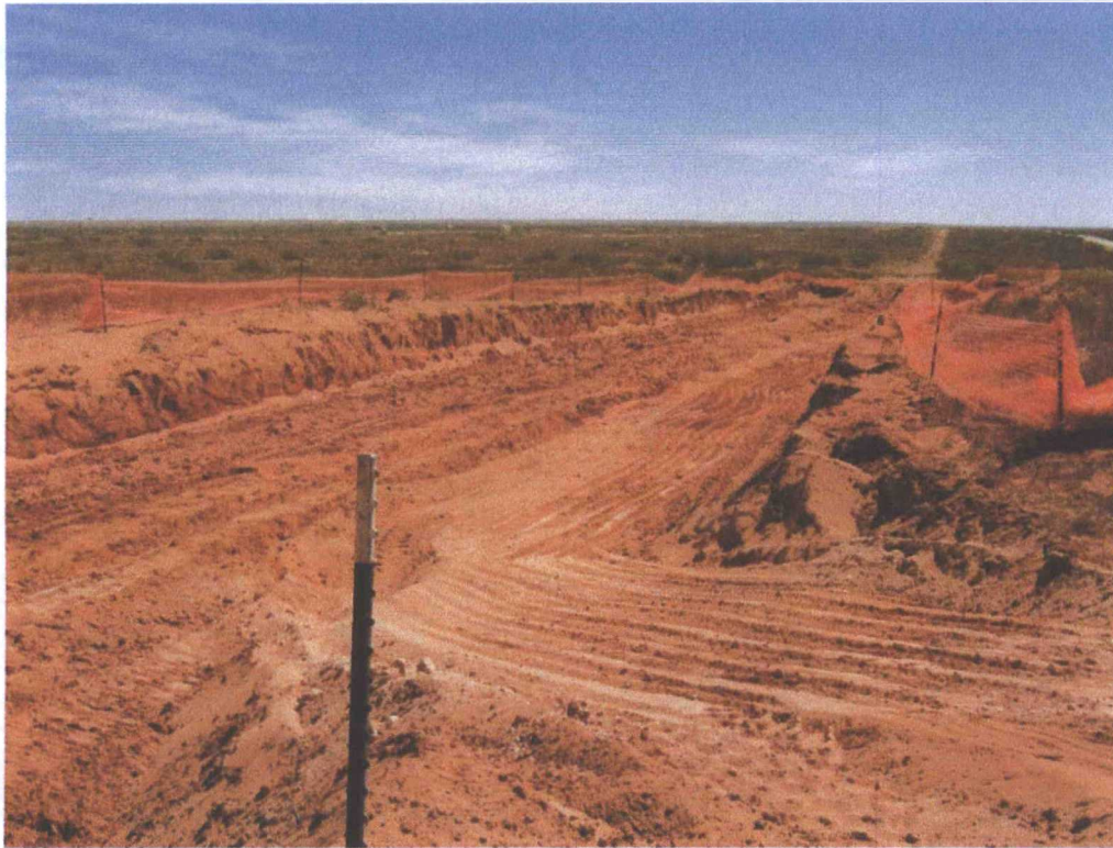
View of Excavation
