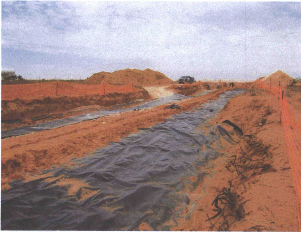
View of Excavation and Liner Installation
