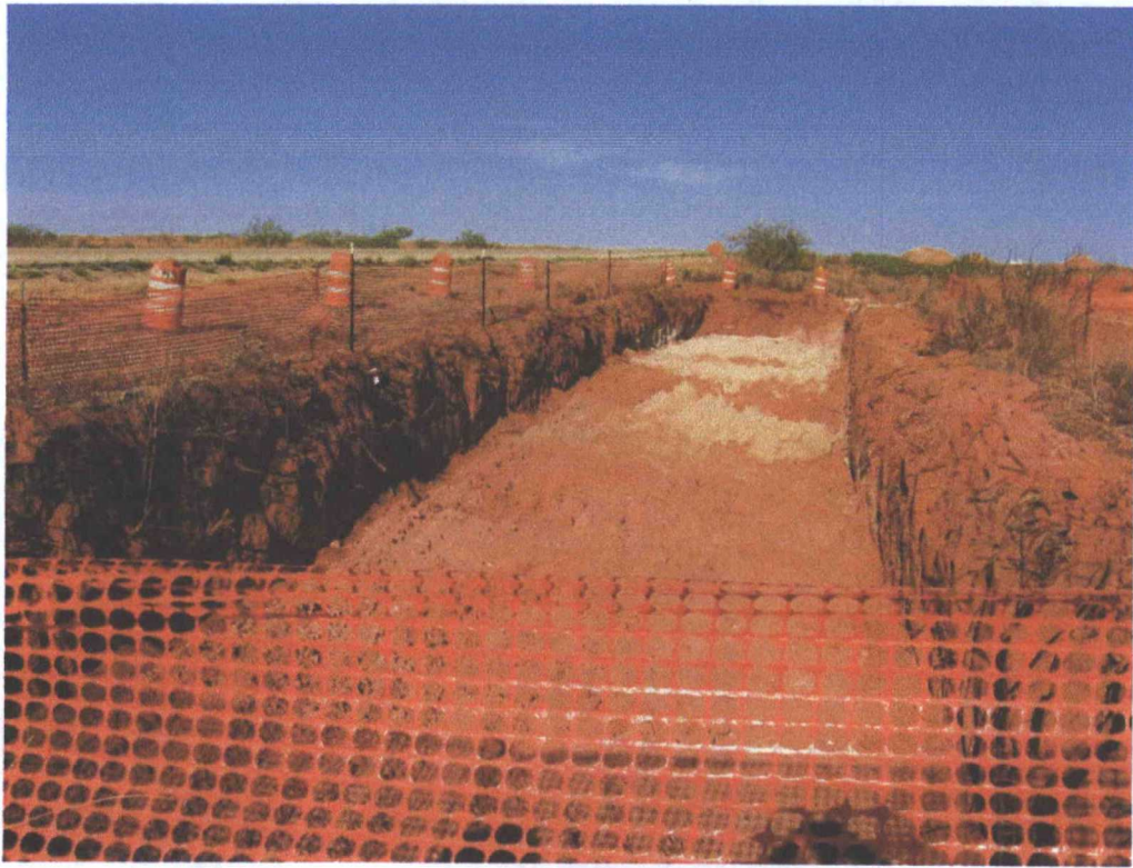
View of Excavation
