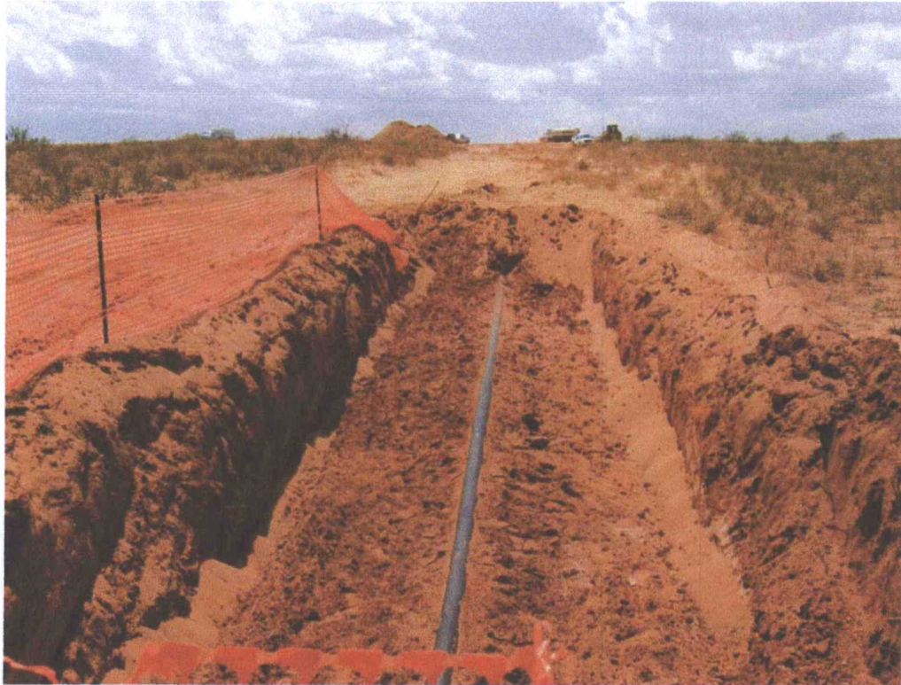
View of Excavation
