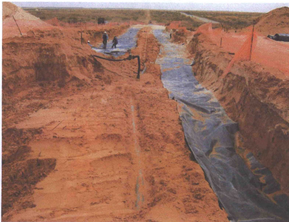
View of Excavation and Liner Installation
