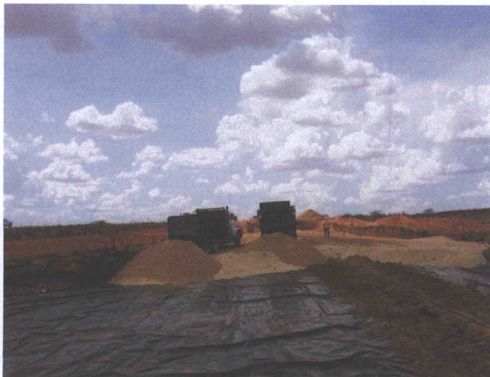
View of Excavation and Liner Installation
