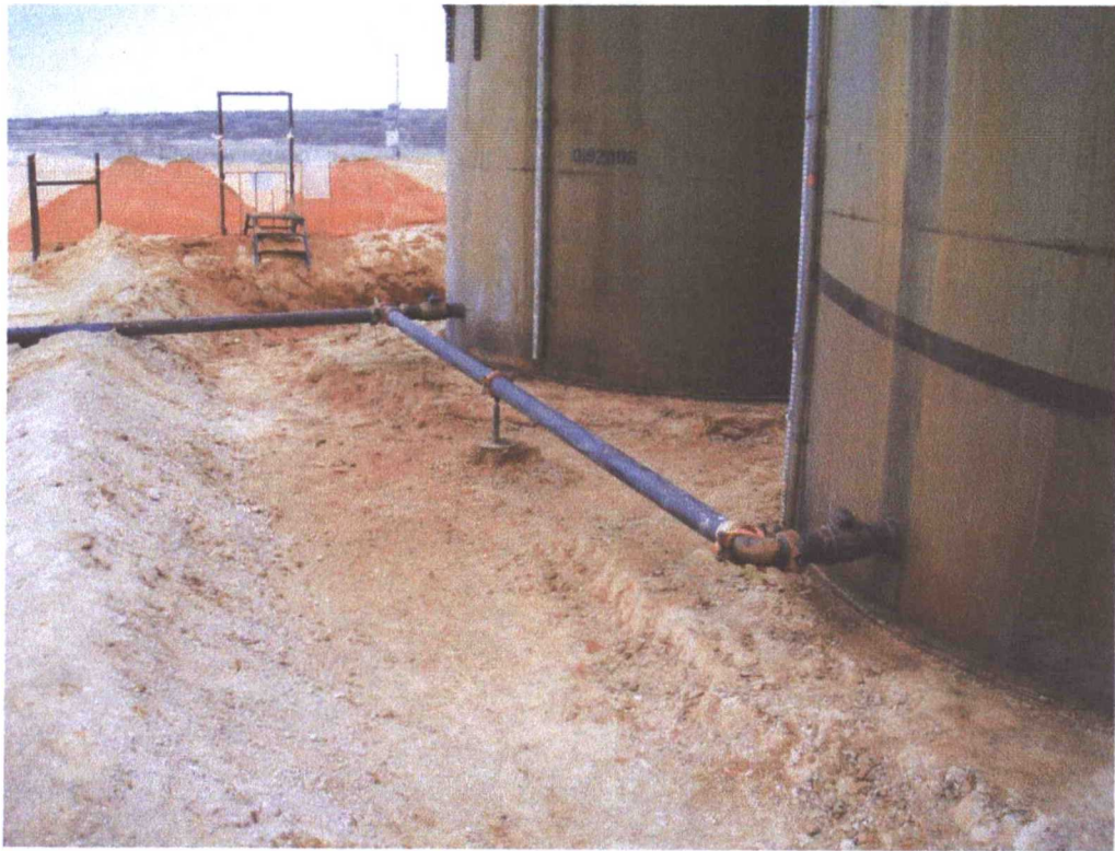
View North – Area of AH-1
