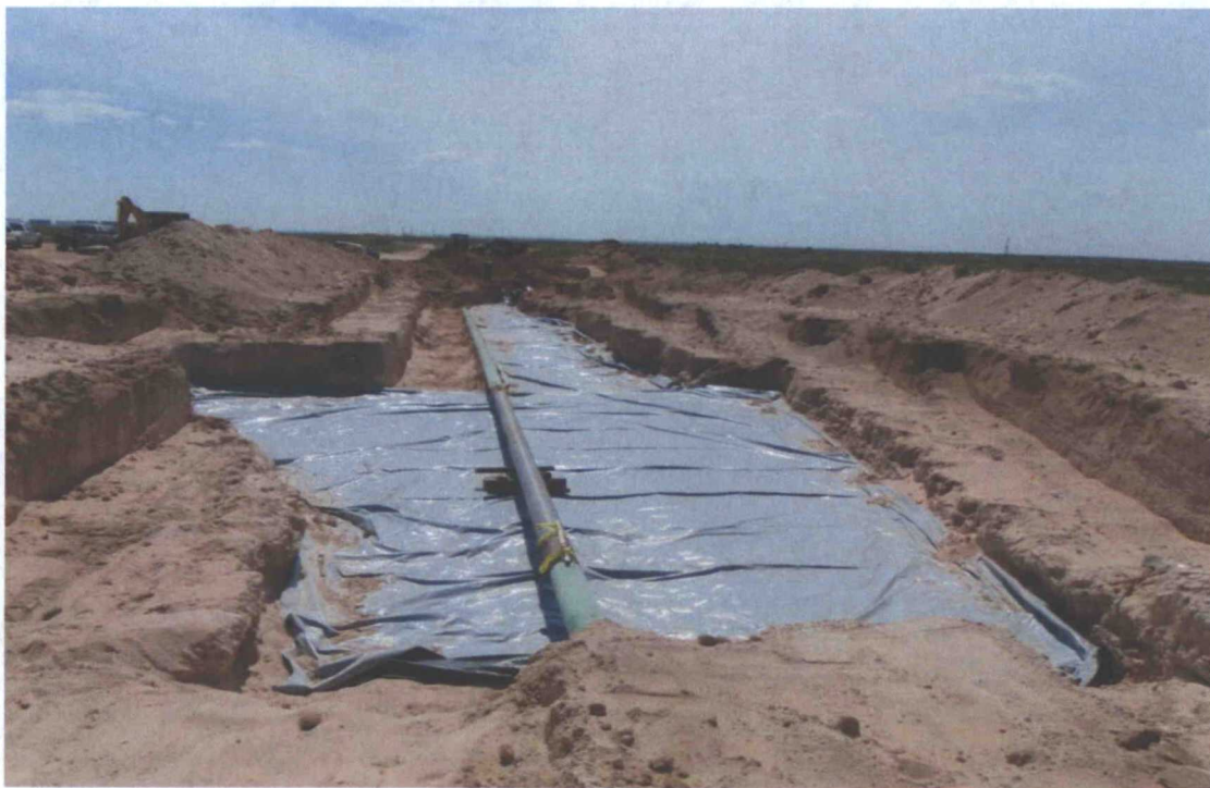
Line #290 (East of Jal South) – Remediation Activities (20-mil Polyurethane Liner)
