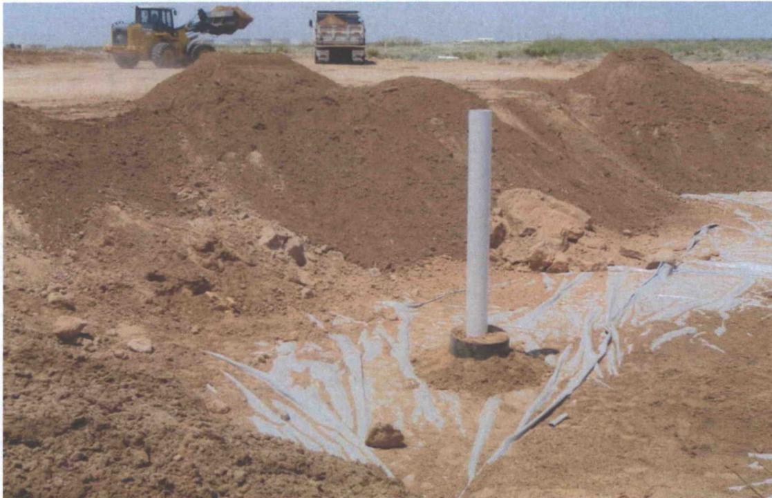
Line #290 (East of Jal South) – Remediation Activities (8" PVC Conduit)
