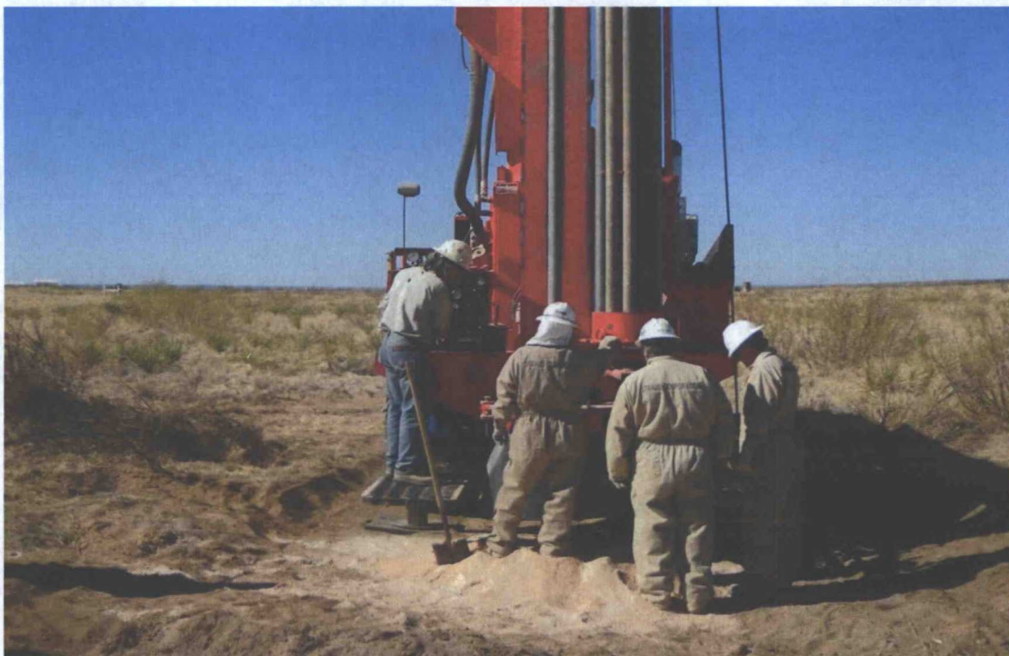
Line #290 (East of Jal South) - Advancement of Soil Boring SB-1
