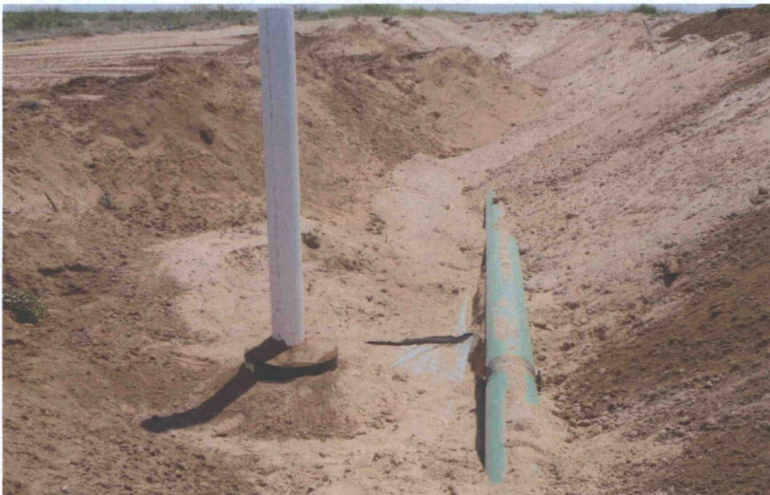
Line #290 (East of Jal South) – Backfilling Activities (8" PVC Conduit)
