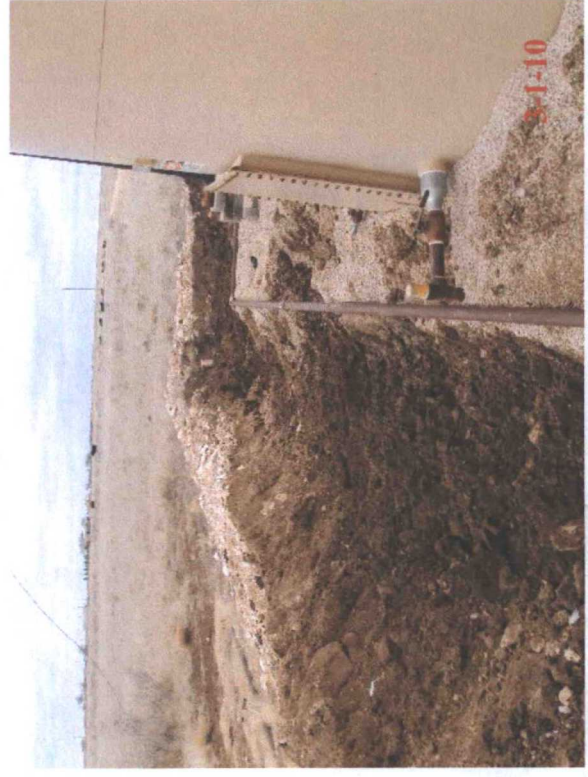
East side of battery after excavation of impacted soil.
