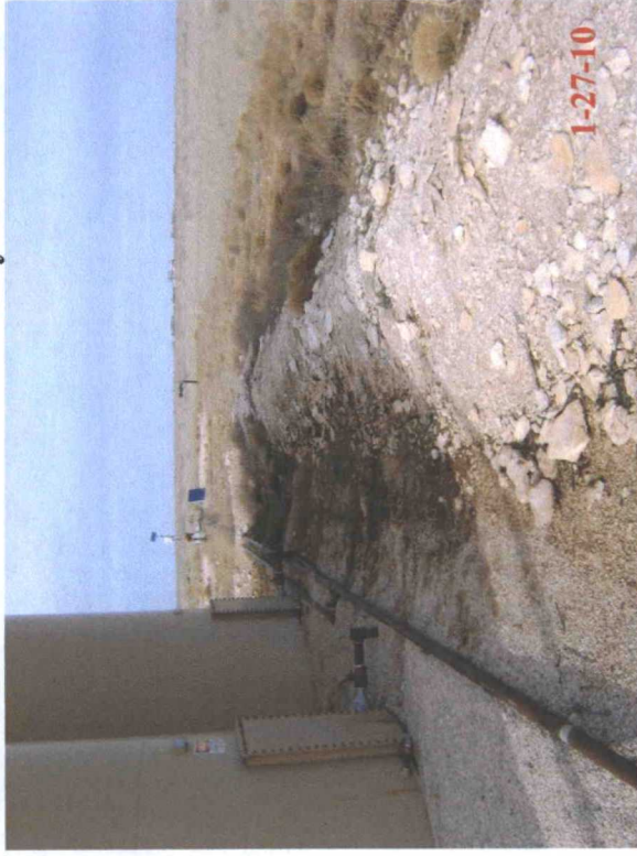
East side of battery before excavation of impacted soil.
