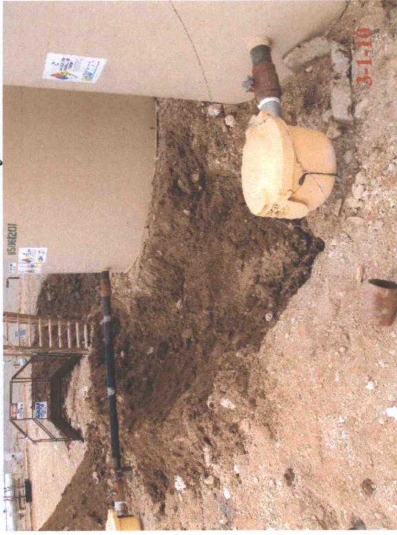
West side of battery after excavation of impacted soil.
