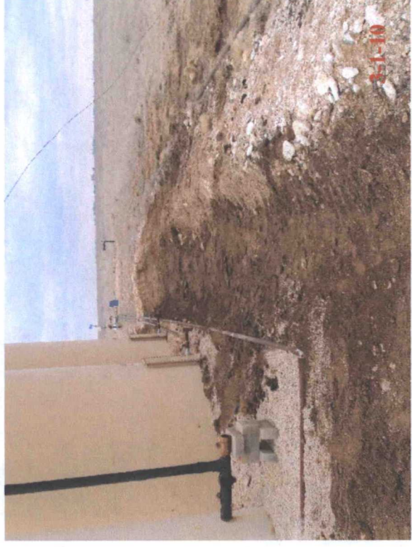
East side of battery after backfill of remediated soil.
