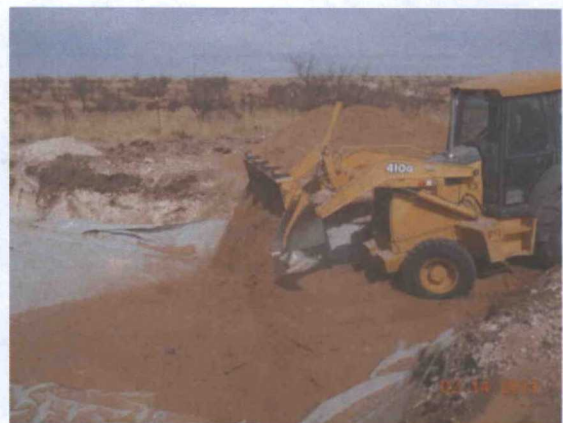
Padding on top of Poly liner with sand, facing north
