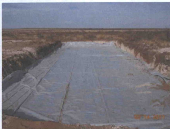
Poly liner installed, facing west
