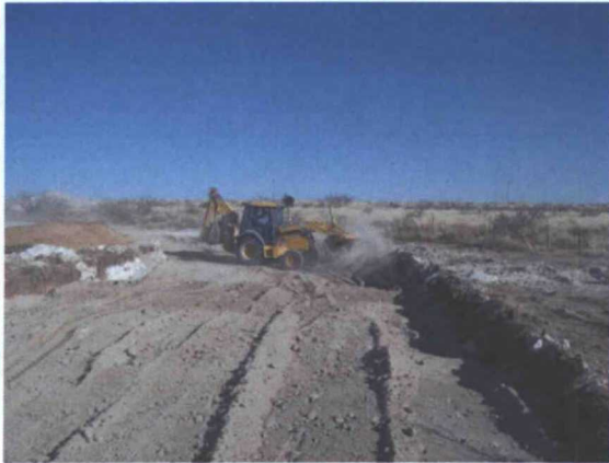
Backfilling excavation, facing east
