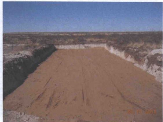
Excavation with sand padding, facing west
