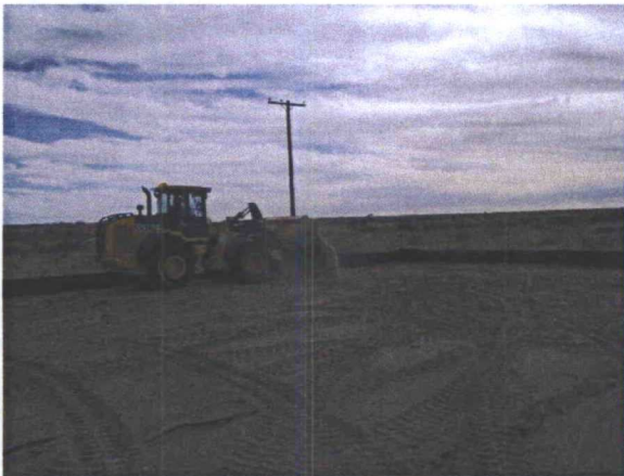
Spreading soil with amendments, facing southwest
