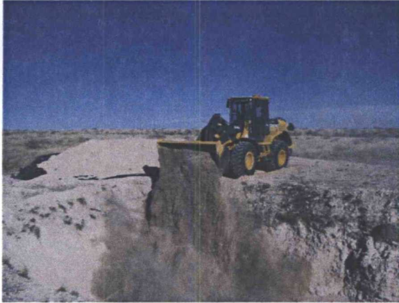
Backfilling excavation, facing northwest
