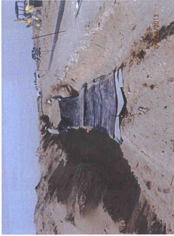
Installing the 20-mil reinforced poly liner, facing west
