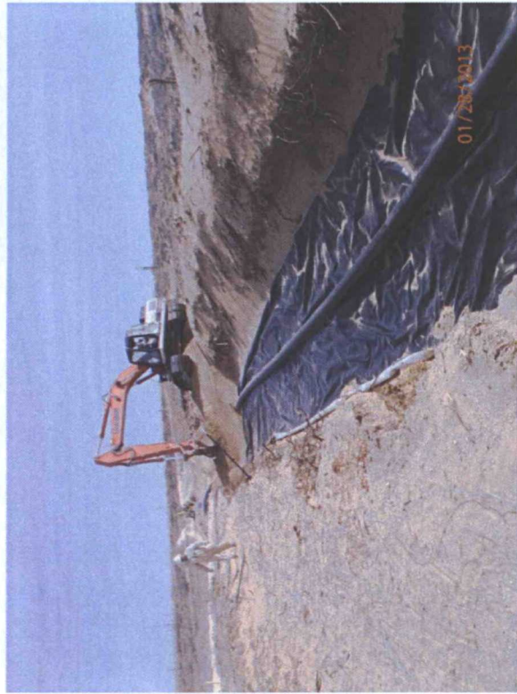
Backfilling above the liner, facing east
