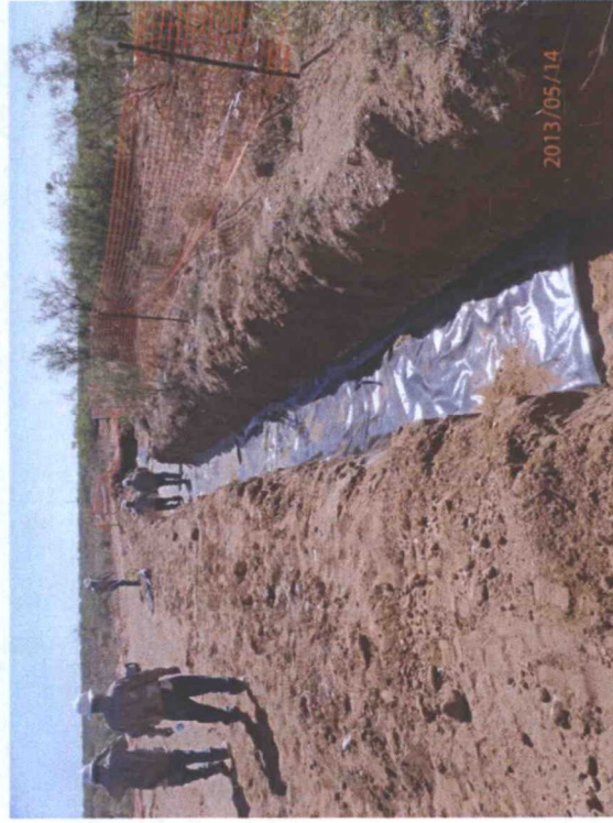
Installing liner, facing east
