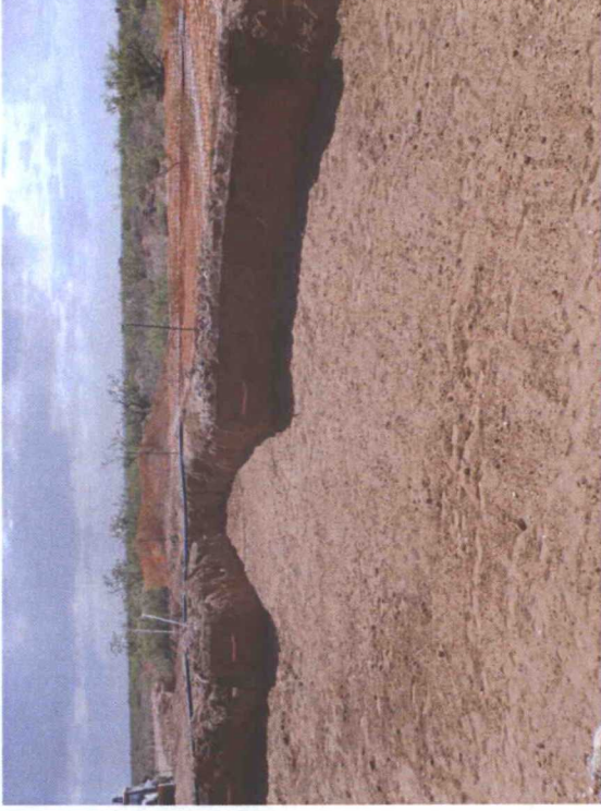
6 inch sand pad completed, facing east
