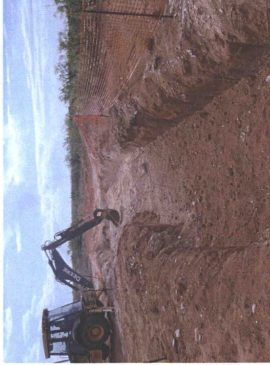
Backfilling the site with caliche, facing east
