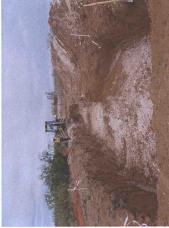
Excavating for liner installation, facing west
