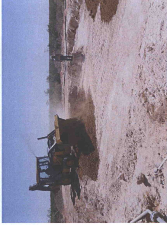
Backfilling the site with topsoil, facing east
