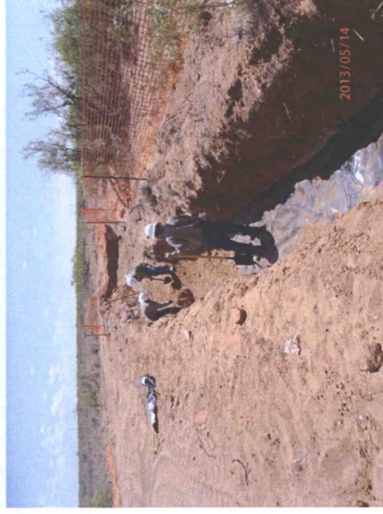
Installing 6 inch sand pad, facing east
