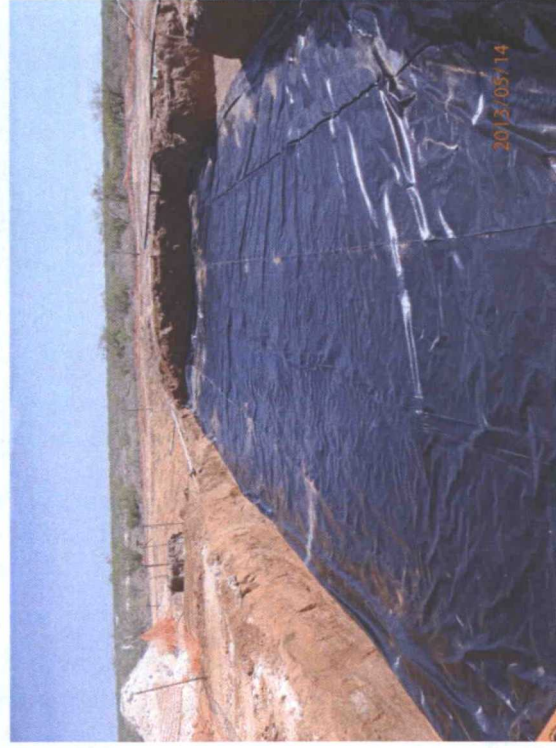
Liner installation completed, facing north
