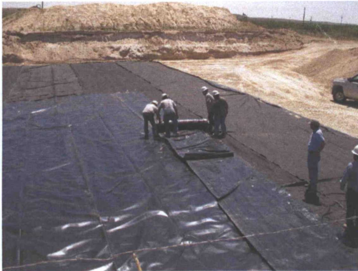
Laying down the double liner
