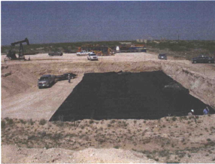
Laying down the first liner
