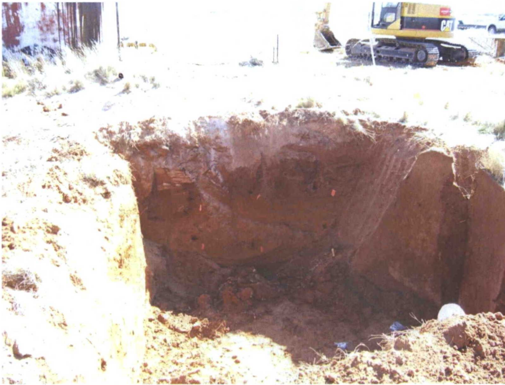
Photograph of the BGT removal and sample locations at Drip Tank #106.
