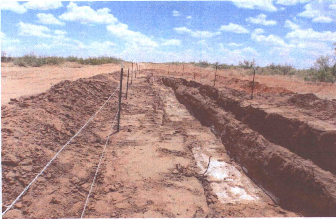
Trunk "M" (King Road) - Excavation
