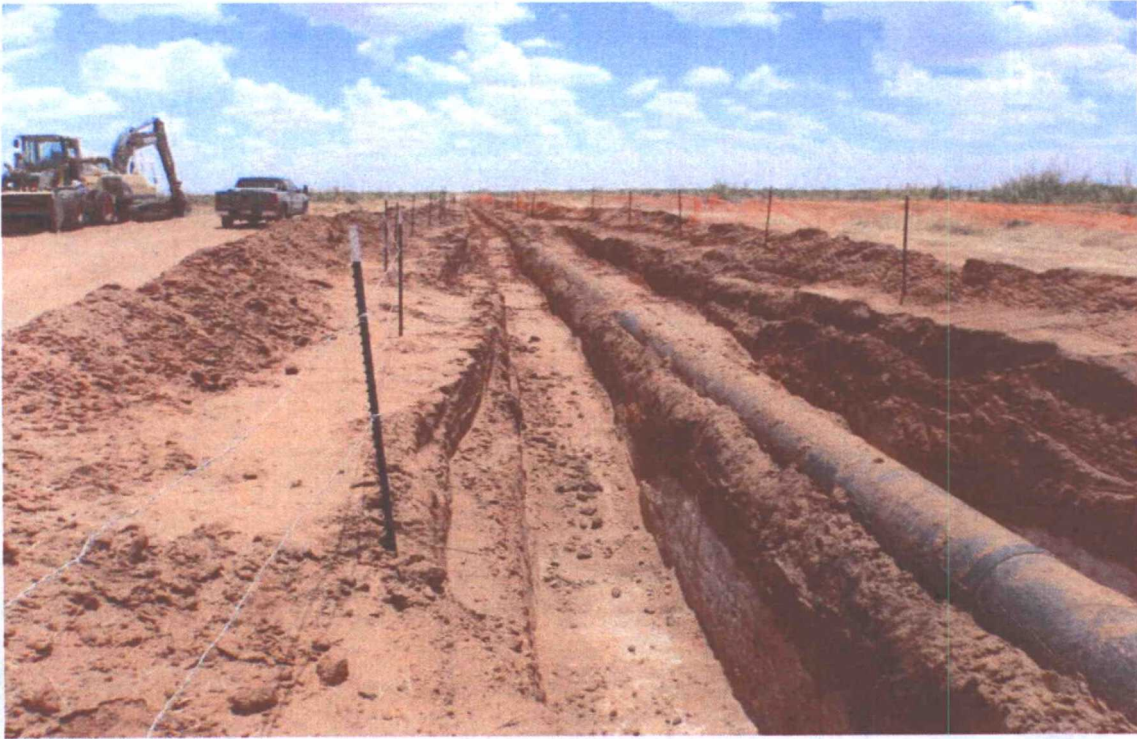
Trunk "M" (King Road) - Excavation
