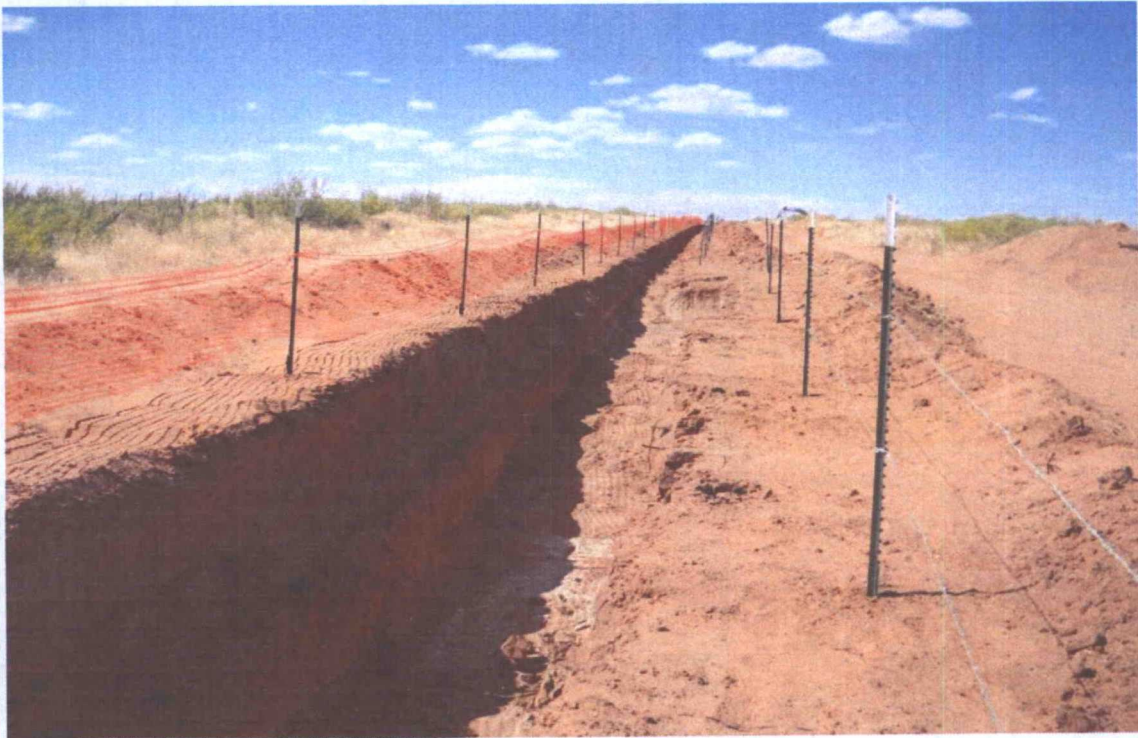
Trunk "M" (King Road) - Excavation
