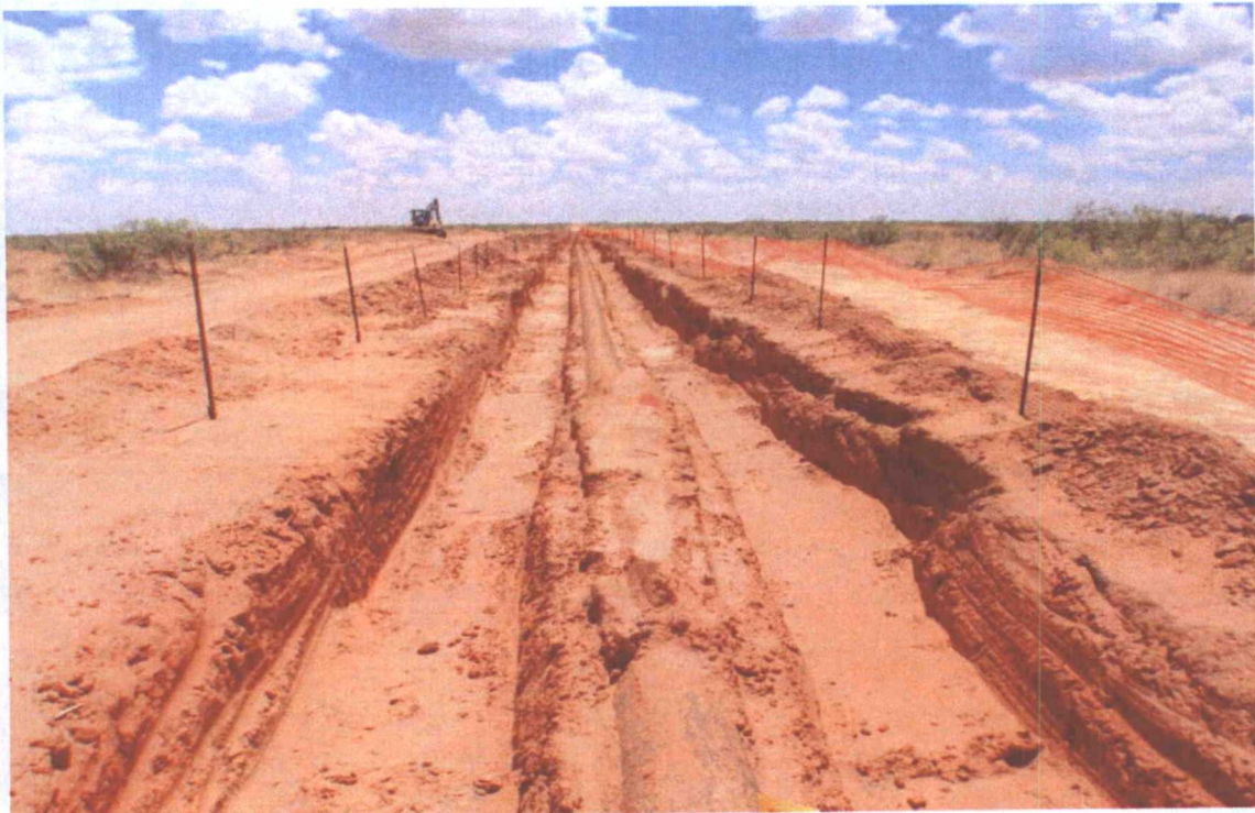
Trunk "M" (King Road) - Excavation
