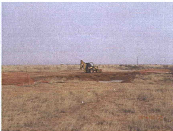
Backfilling and contouring the site, facing southeast 2/25/2014
