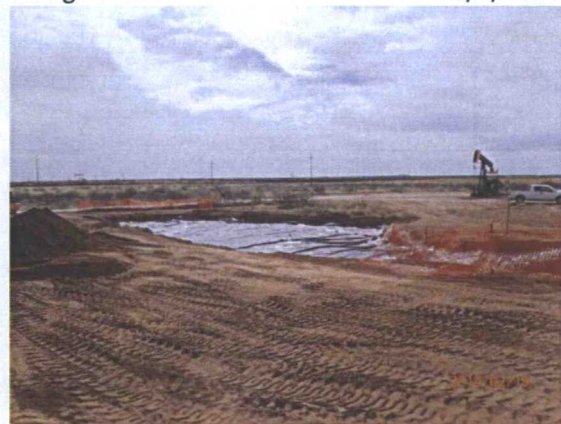
20-mil liner installed in Area 3, facing southwest 2/19/2014
