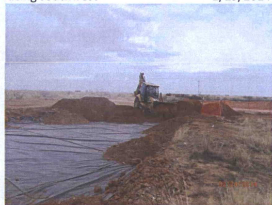
Backfilling above the liner with imported topsoil, facing southeast 2/24/2014
