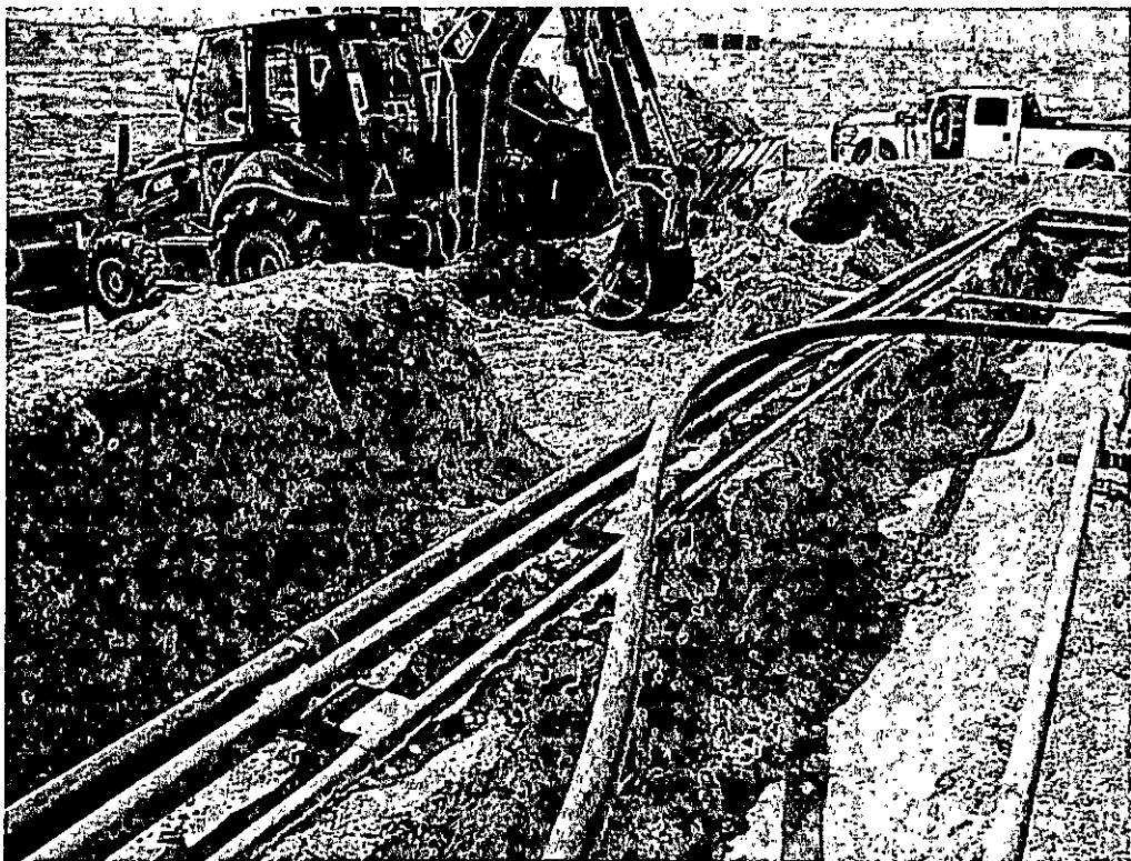
South end of tank battery excavation depth approximately 1.0' bgs
