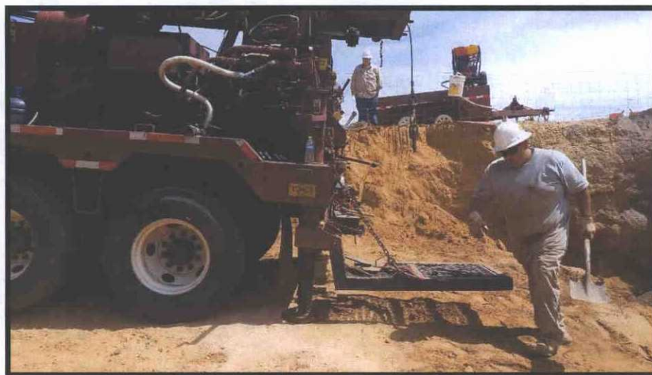
Photo 4: Leveling the CME-85 drill rig within the excavation, concrete pads were used to support the hydraulic jacks.
