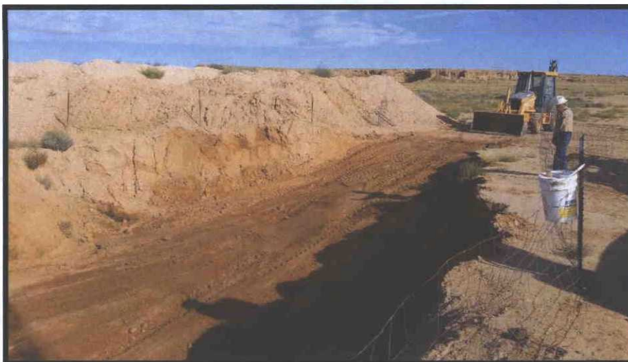
Photo 3: Constructing the ramp and pad for the installation of SB-6 within the existing excavation.
